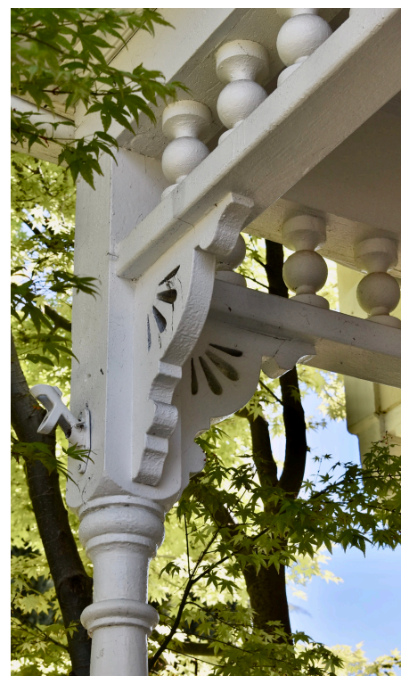
Bottom row: Porch balusters and sunburst brackets.
