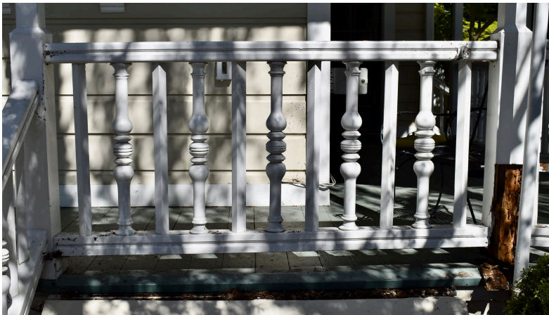
Four photos of the rear addition, including a detail of the railing. All of this fabric dates to 1995 or 1999.
