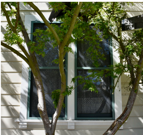
At left: Paired double-hung windows on the south side of the original first story of the rear block of the house.
