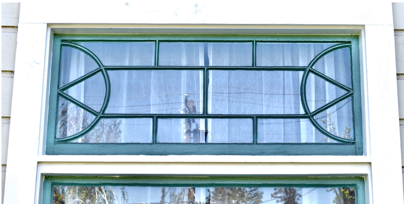
At right and below: Fixed window with transom and panel in the first story bay window.
