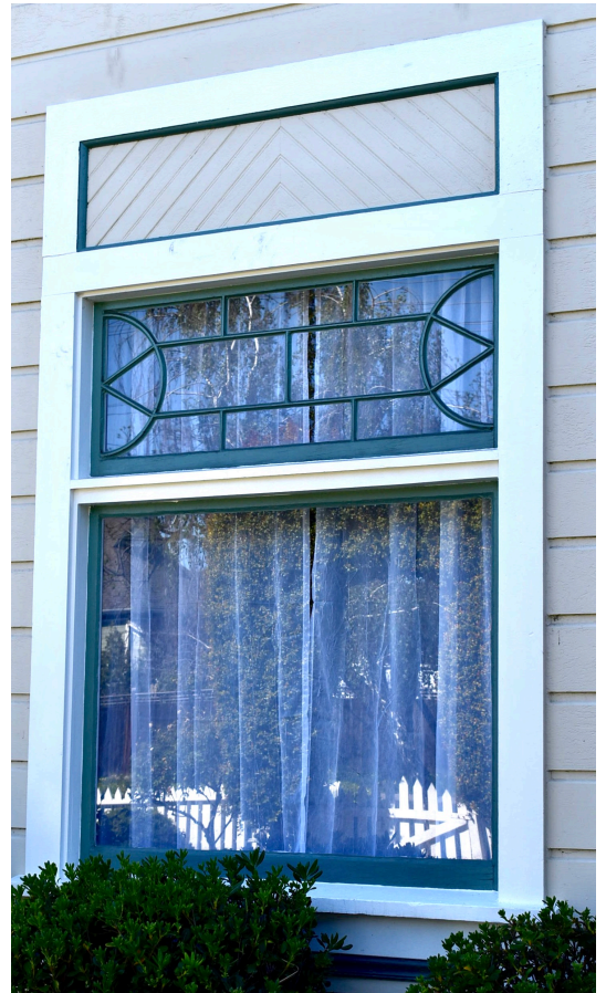
At right and below: Fixed window with transom and panel in the first story bay window.
