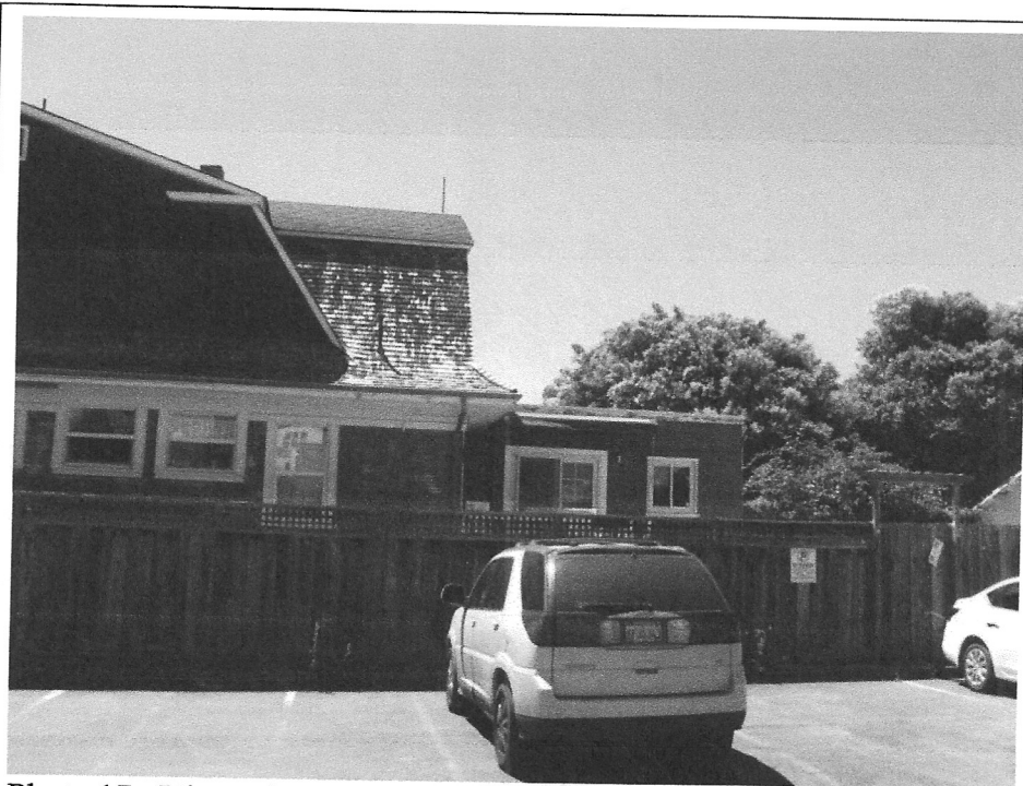
Photo 17: View of rear portion of the northern façade.
