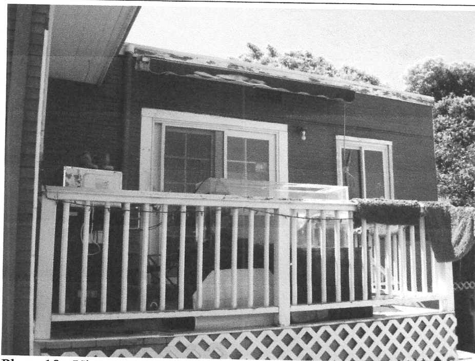
Photo 18: View of the rear addition from the north.
