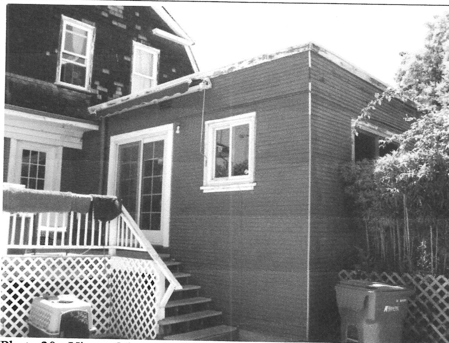
Photo 20: View of the rear addition from the northwest.
