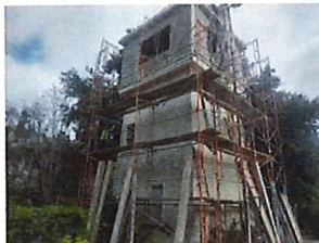
Repairs to Harris Lass
