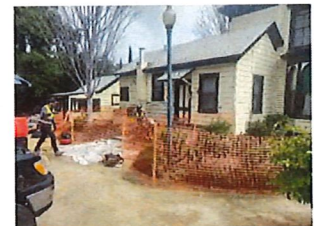
Repairs to Harris Lass
