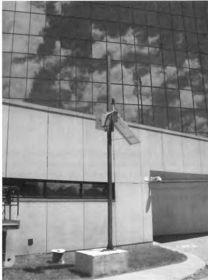
Each noise monitoring station will include a noise sensor, a digital noise logger, and a cellular modem for automatic remote data transmission (24/7). Additional information about the Seti-Media noise monitoring stations may be found in the appendix.
