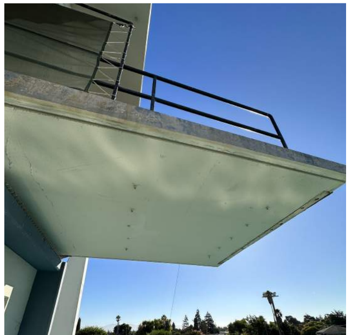
Image 28: Diving Platform in Tower
