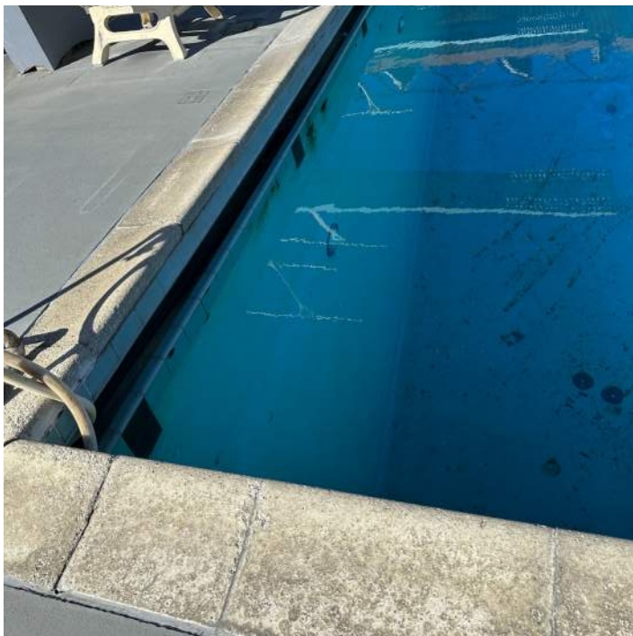
Image 17: Diving Pool Coping Stones
