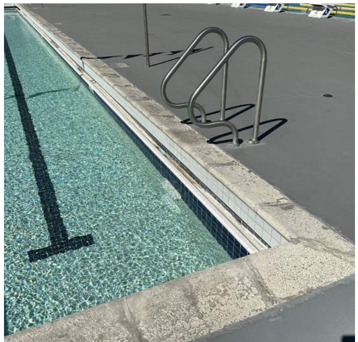
Image 12: Instructional Pool Coping Stones
