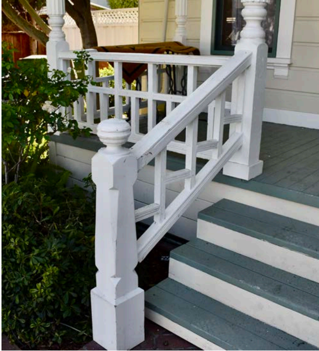
Front porch: Newel posts, balusters, railings, deck, and steps.
