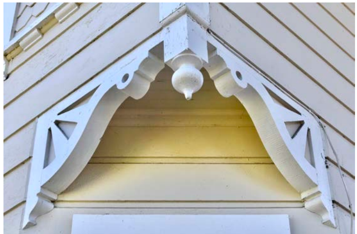
At right: Sunburst brackets with knob pendant in the corner of the bay window.
