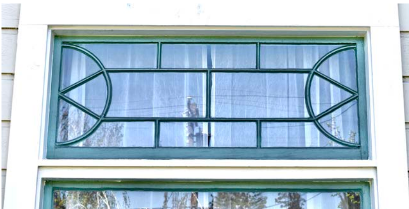
At right and below: Fixed window with transom and panel in the first story bay window.
