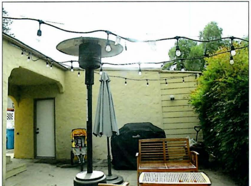
Photo No: 100_2712; View: Arcaded Wing Wall interior view & N side elevation of garage. Photo Date: Sept., 2020; Camera Facing: SSE.
