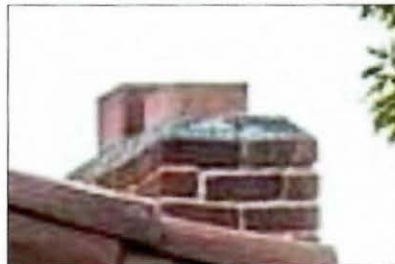
Elaborated Chimney Top
