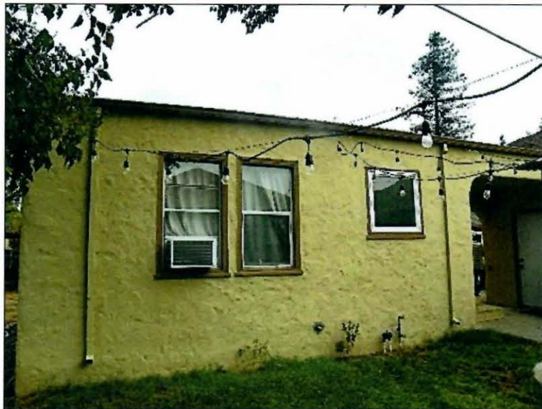
Photo No: 100_2701; View: Rear Façade. Photo Date: Sept., 2020; Camera Facing: E.
