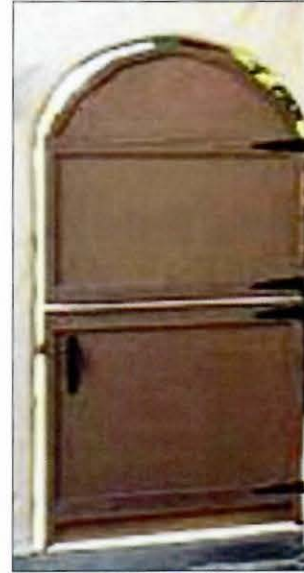
Top: Photo No: 100_2699; View: Arcaded Wing Wall door (arched solid wood plank with iron strap hinges); Photo Date: Sept., 2020; Camera Facing: WSW.
