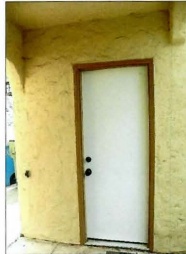
Photo No: 100_2716; View: Garage Man-door; Photo Date: Sept., 2020; Camera Facing: SE.
