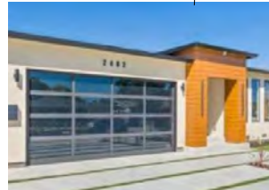
FRONT PORCH WOOD SIDING MATERIALS
