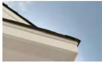
James Hardie Soffit Fiber Cement Vented Smooth Panel painted black satin finish ZK10 FASCIA JAMES HARDY - WITH ROYAL MOLDING
