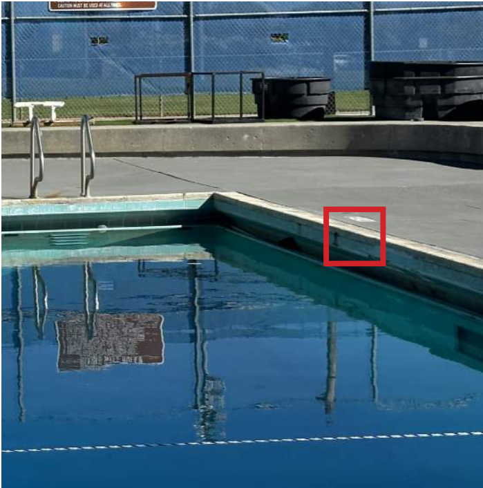
Image 19: No Waterline Depth Marker
