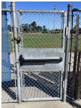
EXISTING CHAINED EXIT
