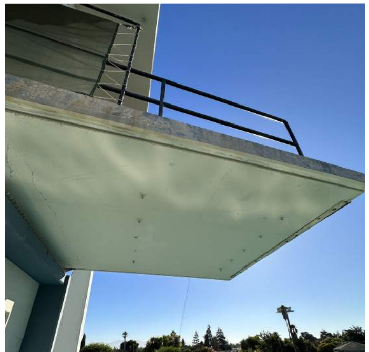
Image 28: Diving Platform in Tower
