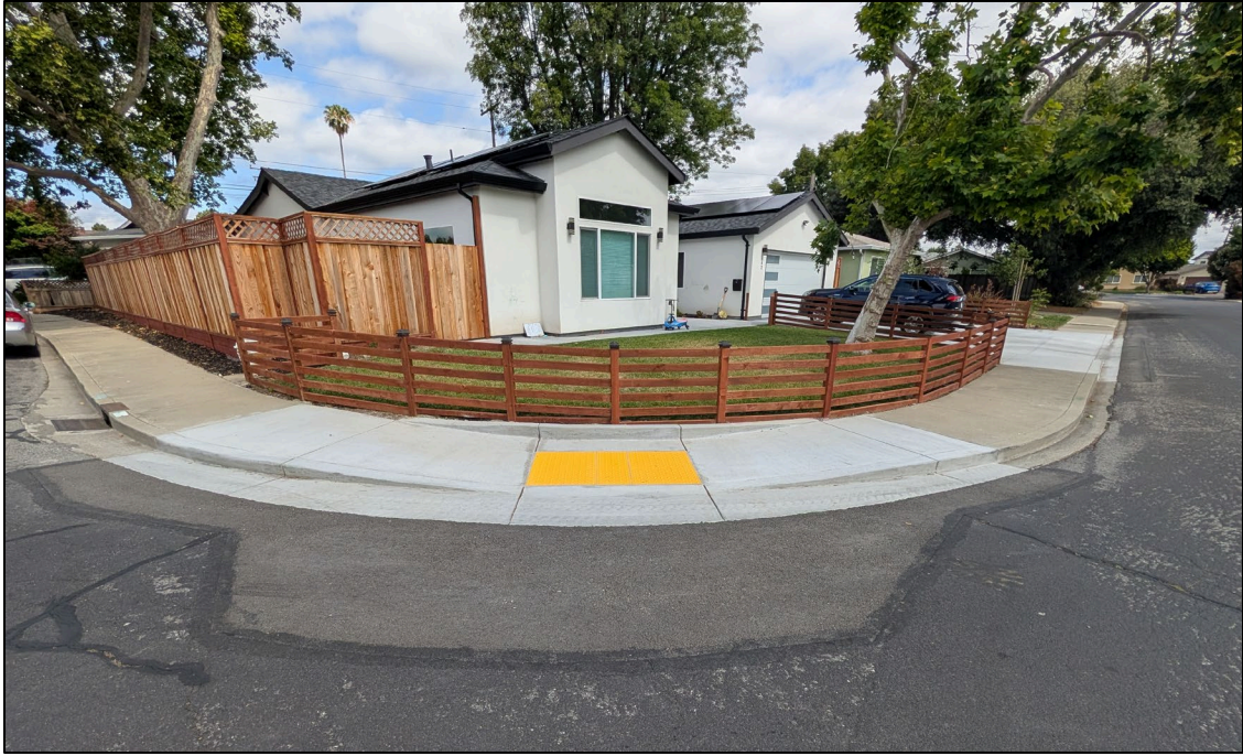
Curb Ramp Improvement
