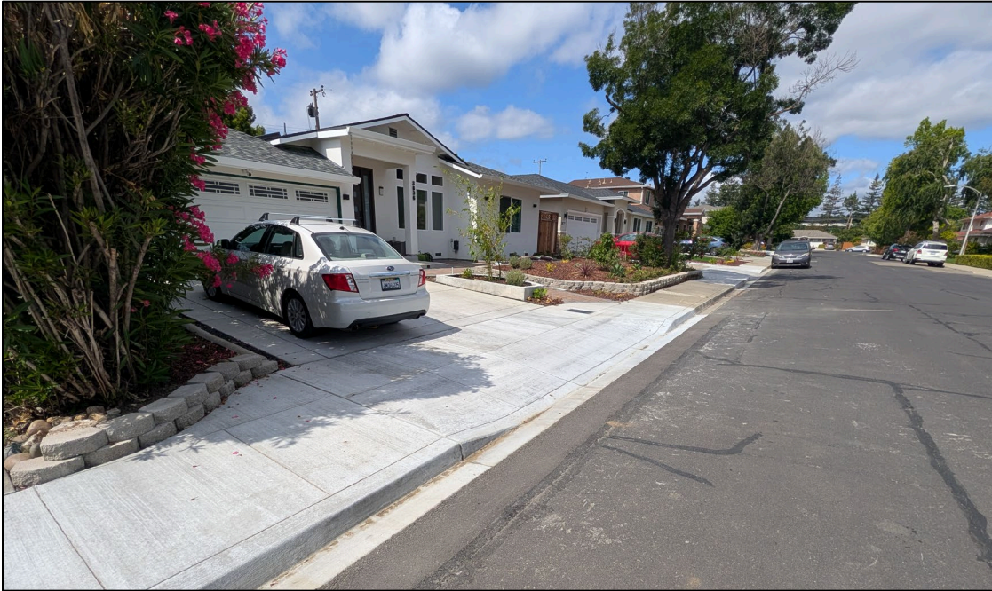
Driveway Approach and Sidewalk Improvement
