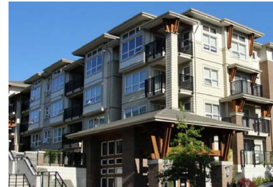
5.6.1.4 - Variation in Roof Lines
