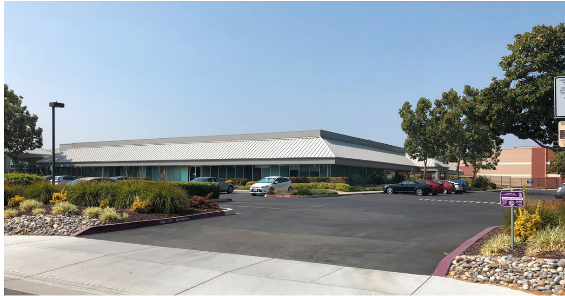
Low-density Office Building on Patrick Henry Drive
