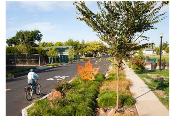
5.2.3.8B - Stormwater Planters in Bulbout
