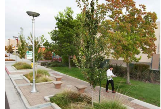
5.2.3.8A - Stormwater Planters in Pedestrian Zone
