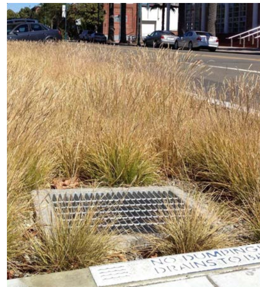
Street-level Stormwater Drain
