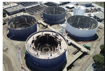
Digester Facilities Upgrades
