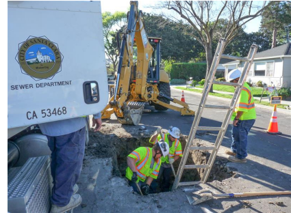
City Crews Repairing Sewer Pipe
