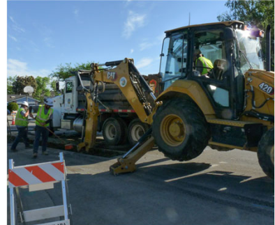
City Crews Replacing Water Main
