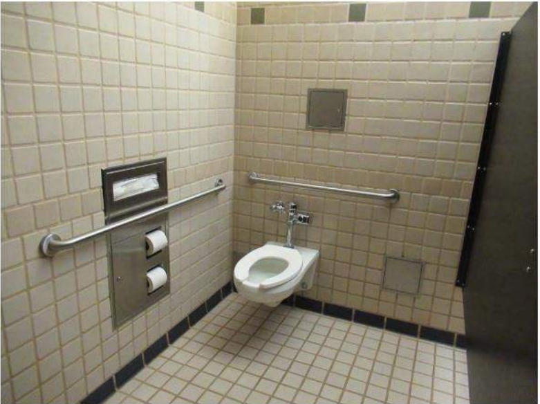
42. Toilets have automatic flush valves.
