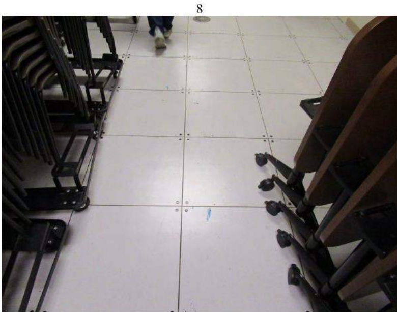
8. Typical raised floor throughout the facility.
