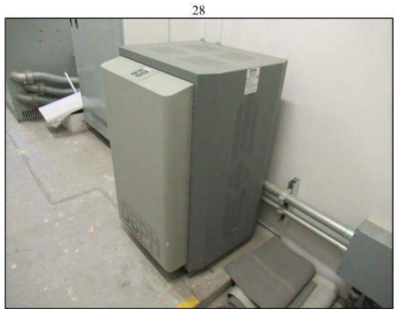
28. An Inverter supplies backup power to emergency egress lighting.
