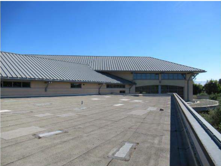
29. Roof membrane over the south roof is a multi-ply with capsheet that is 20 years old.
