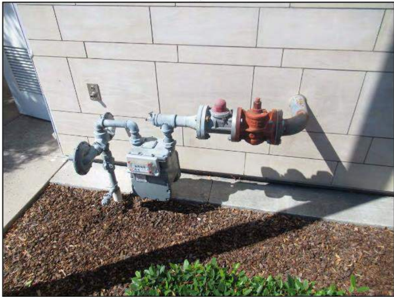
23. Gas service with seismic valve.
