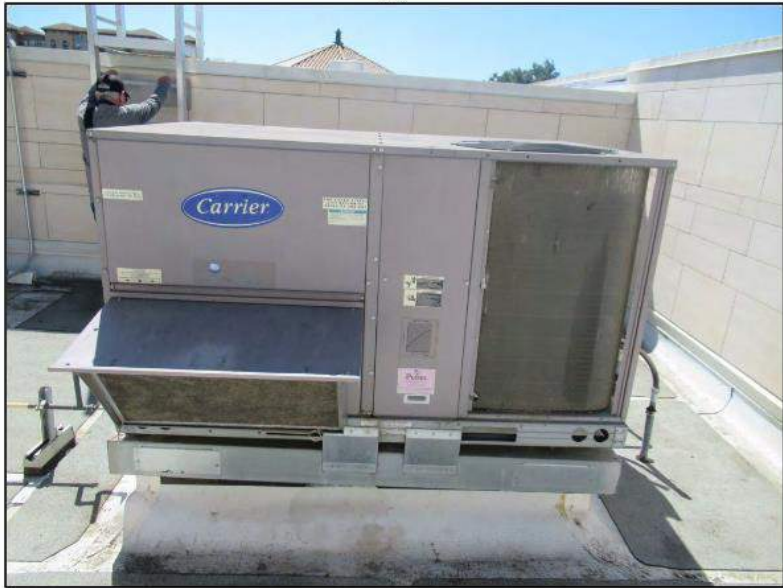
20. One Carrier 5-ton packaged unit on the roof for the community room.
