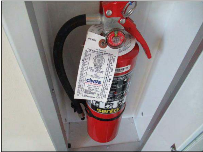
26. Fire extinguishers have current service tags.
