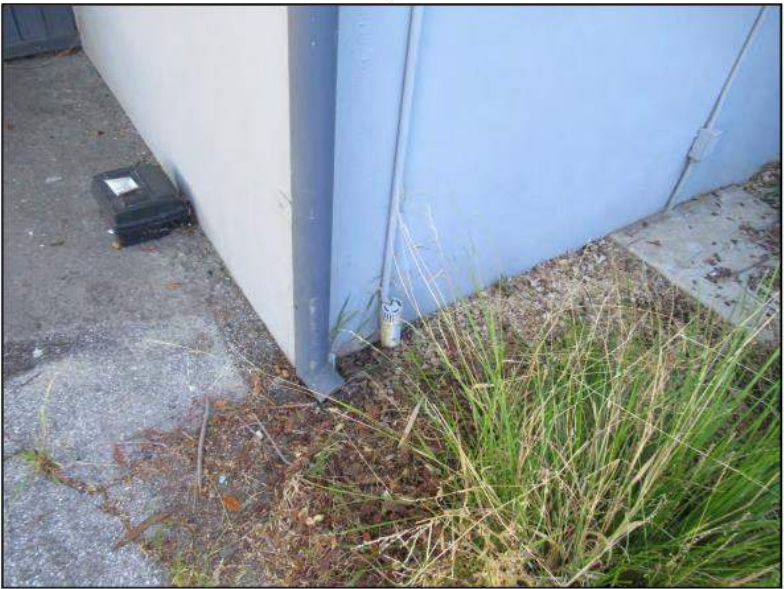
7. Downspouts discharge at grade.
