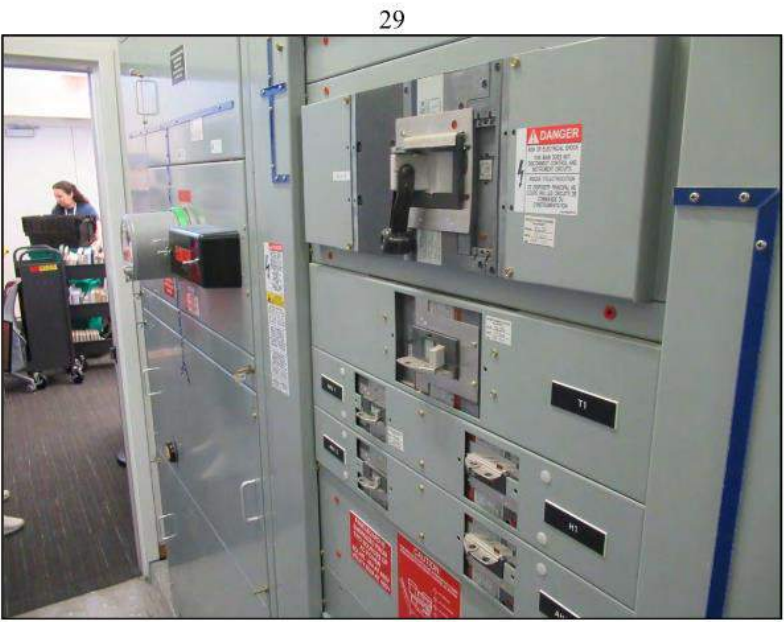
29. View of the 800-ampere main switchboard.
