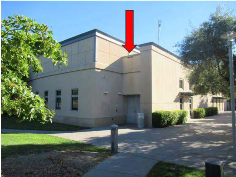
14. View of the southwest corner. Note staining from the roof scupper above door.
