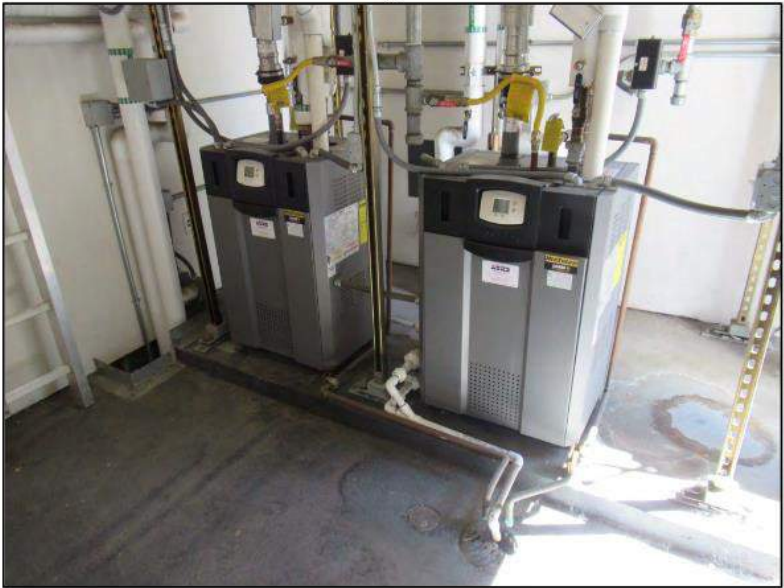
18. Natural gas-fired boilers for space heat.
