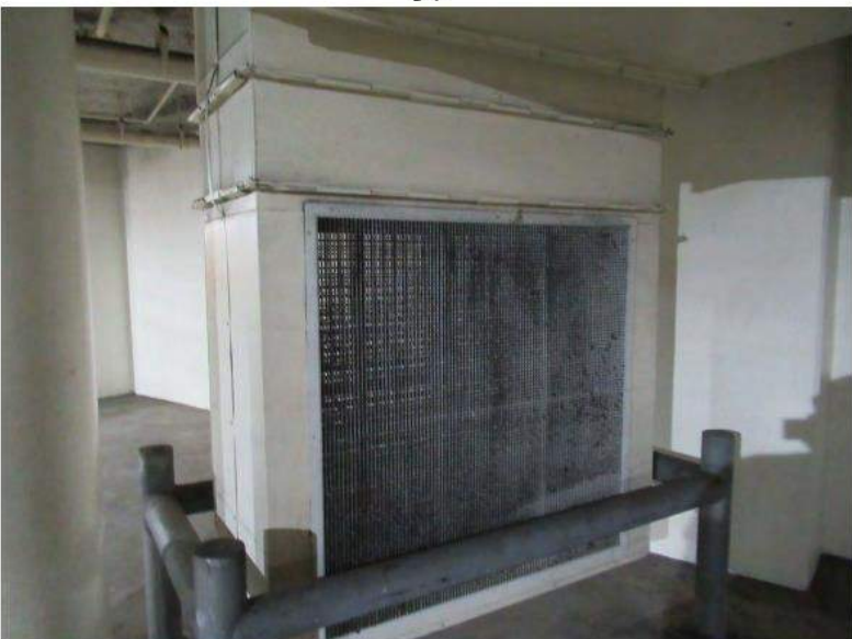
34. Garage exhaust intake.
