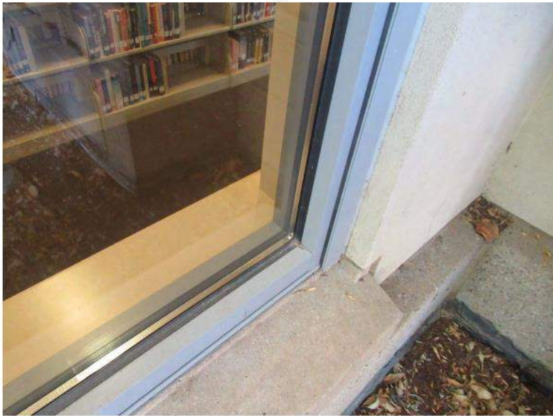
11. Windows are aluminum frame with insulated glazing.
