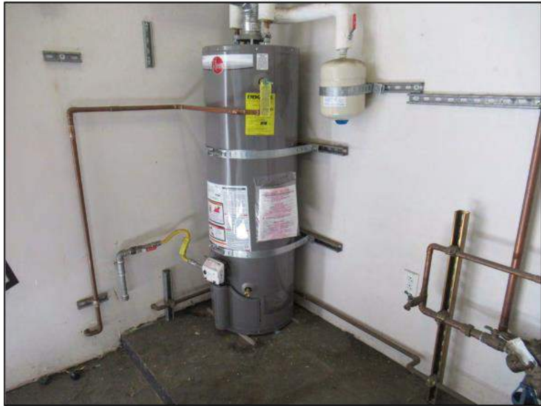
24. Domestic water heater is relatively new.
