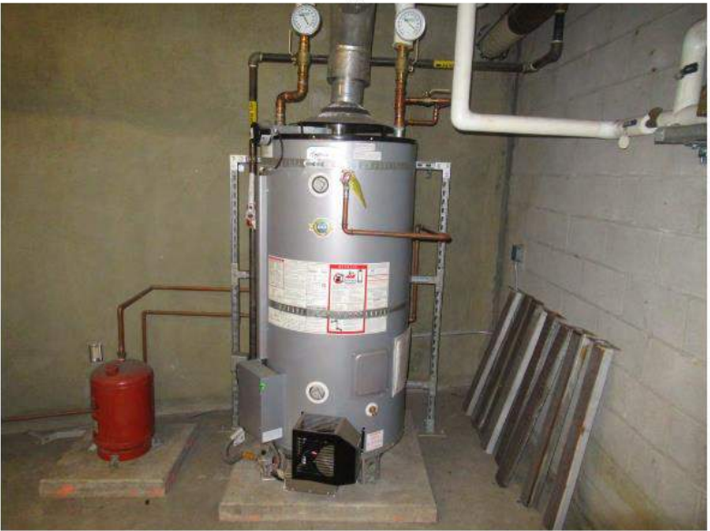
41. American Standard gas domestic water heater.
