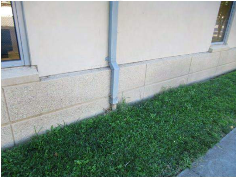
13. Downspouts connect to the underground collection piping.
