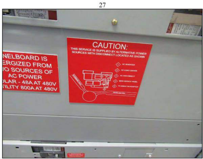
27. The electrical service is supplemented by a solar system.
