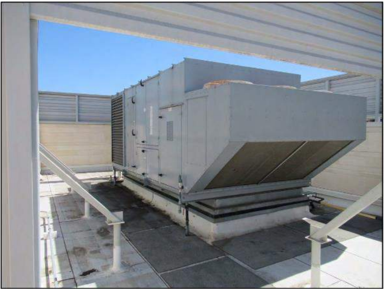
21. One of two 20-ton packaged Airtex units. Number two unit is down for repairs.
