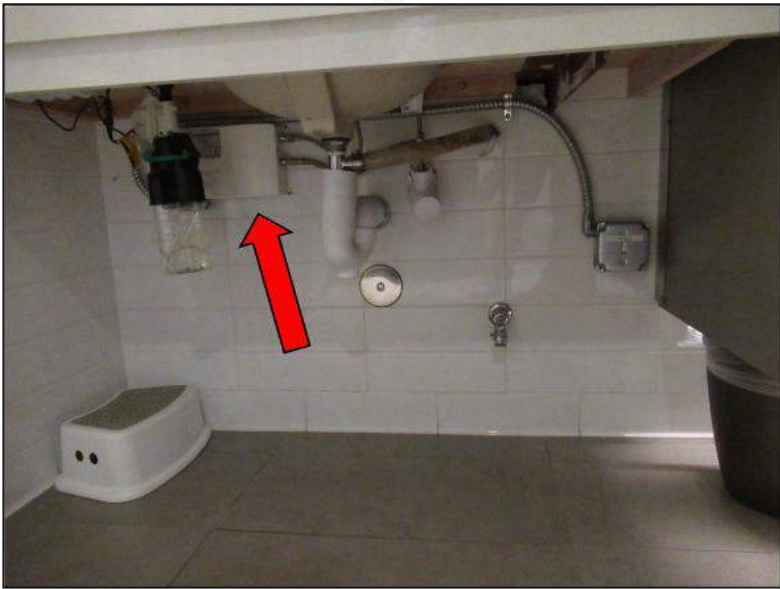
21. Insta-hot electric undercounter water heater.
