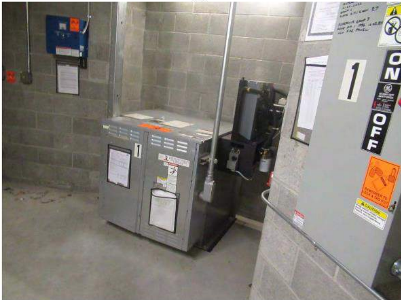
51. One of three hydraulic elevator machines.
