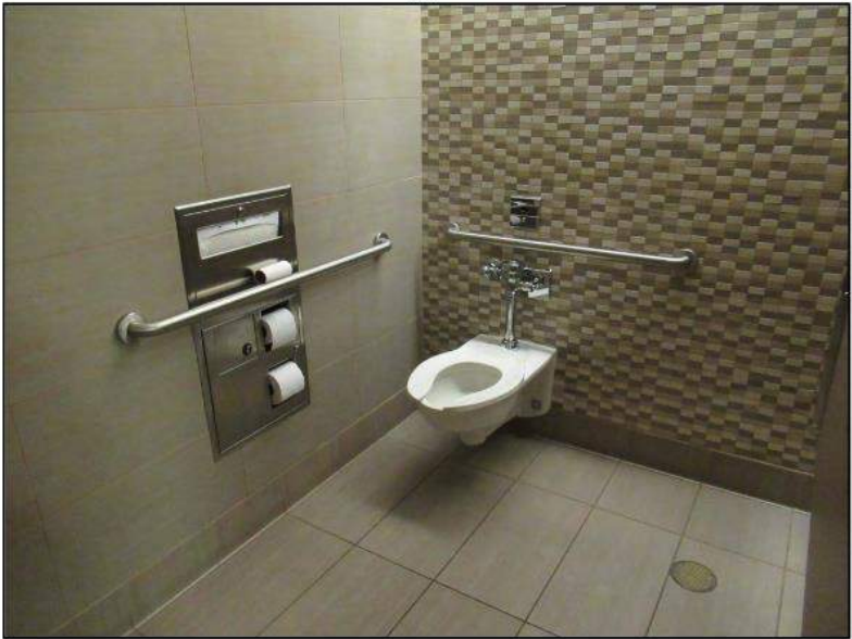
26. Toilets are wall-mounted with automatic flush valves.
