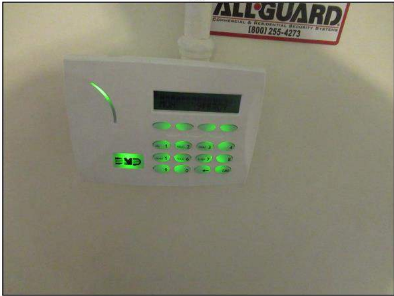
29. Remote fire alarm panel.
