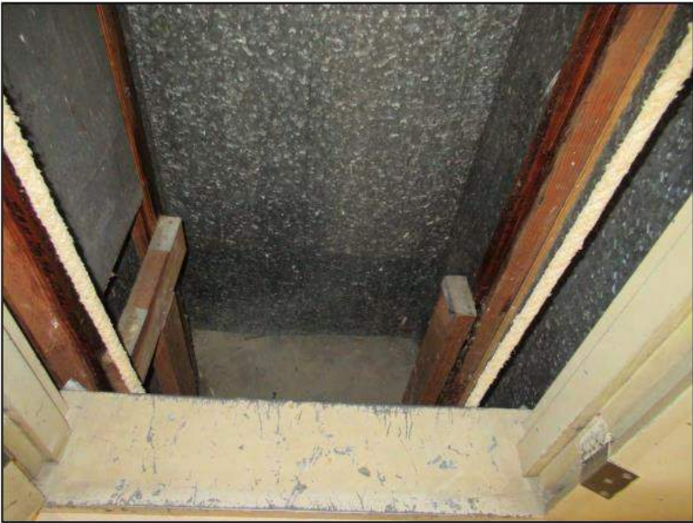
4. Manual dumb waiter to the basement.
