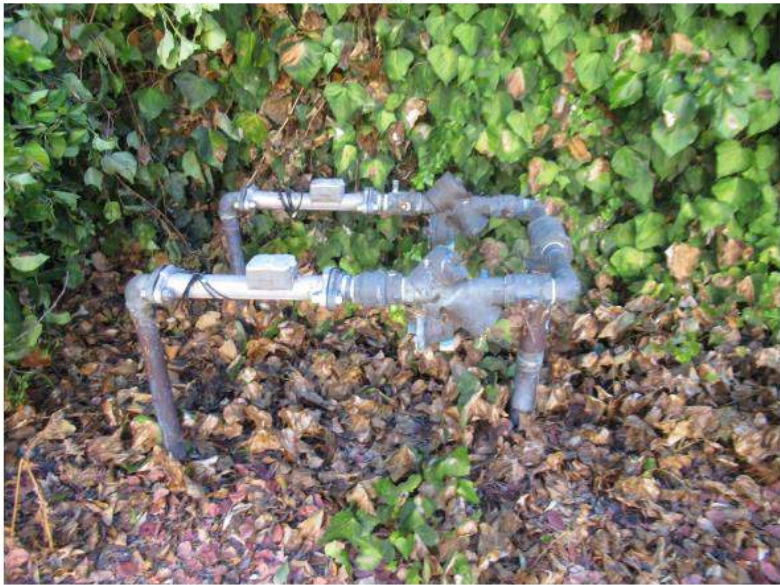
39. Main domestic and irrigation water assembly.
