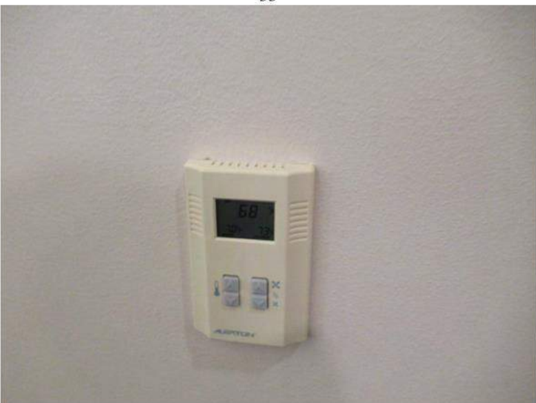
33. Typical Alerton digital thermostat.
