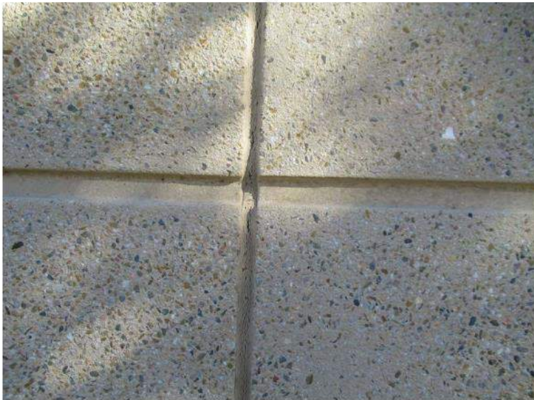
15. Caulking at the precast panel joints is shrinking and needs to be cut out and replaced.
