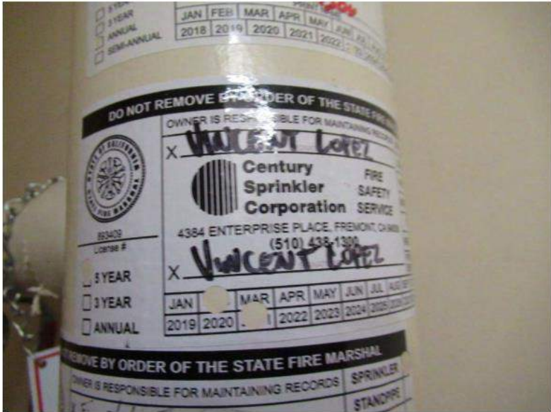
48. The five-year fire sprinkler test label is current.
