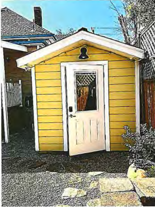
Above: Photo No: IMG_1414; View: “Original” Garage Rear façade and entry door seen from rear yard; Photo Date: 2/6/2026; Camera Facing: WSW.
