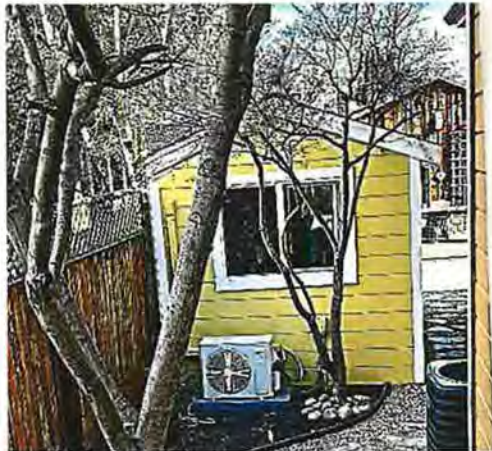
Below: Photo IMG_1431; View: “Original” Garage Front façade, view towards rear yard. Photo Date: 2/6/2026; Camera Facing: ENE.
