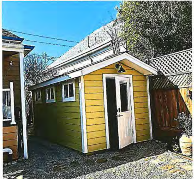
Photo No: IMG_1441; View: “Original” Garage south side-elevation & rear façade; Photo Date: 2/6/2026; Camera Facing: W.
