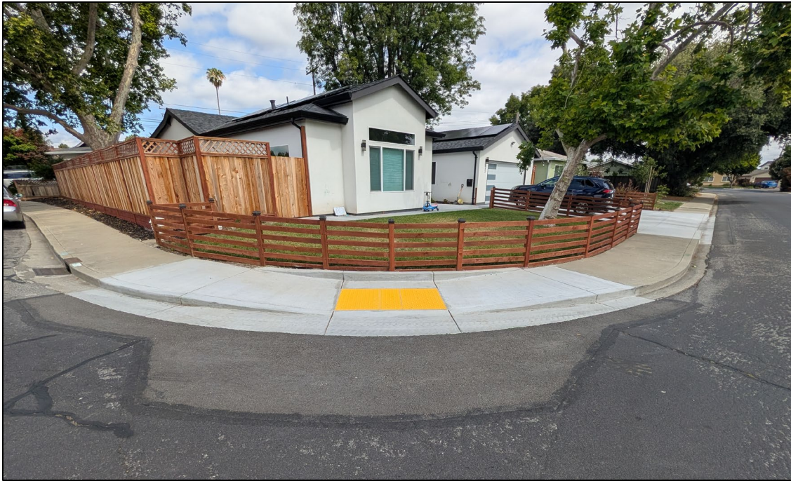
Curb Ramp Improvement
