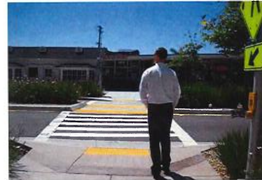
5.2.2.1 - Three-foot Deep Detectable Warning Surface
