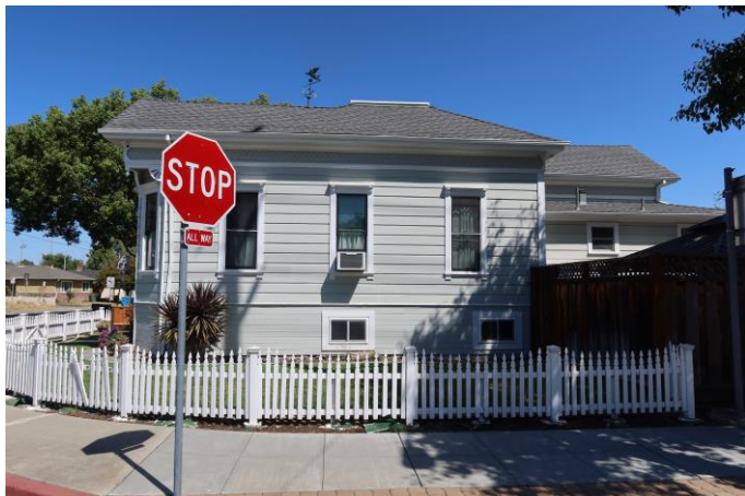
Harrison Street (south) façade.
