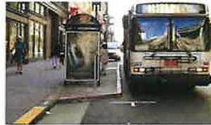
Bus Bulb in San Francisco Source: National Association of City Transportation Officials
