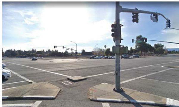
2. FACING SOUTH AT THE CORNER OF SAN TOMAS & MONROE STREET
