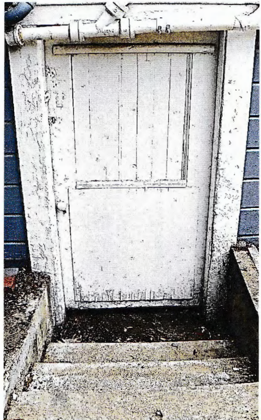
Photo No: 100_3659; View: Basement Entry Door; Photo Date: 8/2/2024
