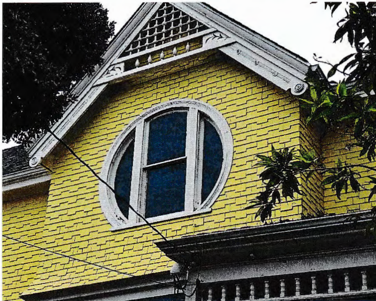
Photo No: 100_3640; View: E side-elevation Gable face with Moon window, Gable screen, carved bargeboards; Photo Date: 8/2/2024; View SW
