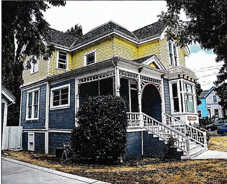
Photo No: 100_3624; View: West side-elevation and partial front façade. Photo Date: 8/2/2024; Camera Facing: N
