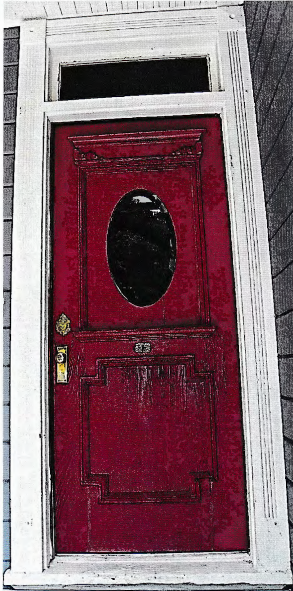
Photo No: 100_3680; View: Front Entry Door, transom & trim Photo Date: 8/2/2024.
