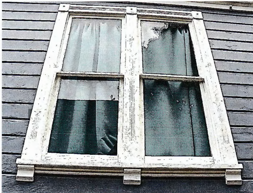
Photo No: 100_3670; View: Typical pair of dbl-hung windows with fluted trin & corner blocks and brackets under the projecting sill; Photo Date: 8/2/ 2024; Camera Facing: W.
