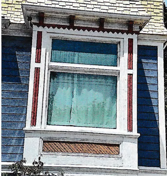
Photo No: 100_3694; View: Front Façade Box Bay; Photo Date: 8/2/2024; View NW
