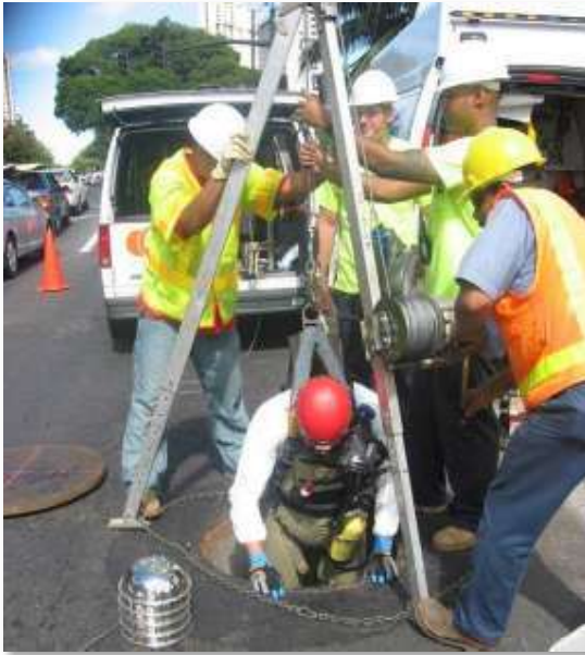
Photo 2-1. Confined Space Entry
