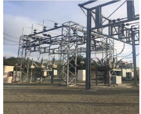
**Project Description** This project reconstructs the Homestead Substation and replaces 60 kV bus work, breakers, old metal clad switchgear with new 12 kV switchgear and transformers. Existing switchgear is 45 years old and obsolete; spare parts are no longer available. Some replacement items are custom built, requiring specialized vendors for procurement that include long delivery timeframes.
