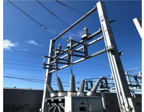
**Project Description** This project installs new 115kV bus structures and related bus switches and breakers at the Northern Receiving Station (NRS). This includes procuring and installing new Breaker 392 and related control panels in the NRS control building with new relays and panels in accordance with current SVP specifications.
