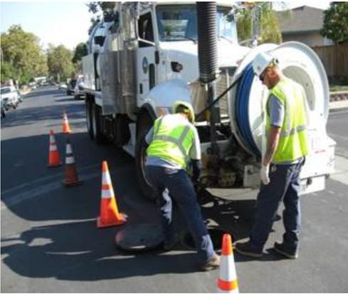
This project funds repairs to the sanitary sewer system that were identified by cleaning and CCTV inspections of the sewer collection system funded by the Sanitary Sewer System Condition Assessment project also in this program. The assessment of the system is on a four-year cycle and deficiencies will be rated based on accepted industry ratings systems, namely the National Association of Sewer Service Companies (NASSCO) system. The most serious deficiencies will be prioritized each year.
