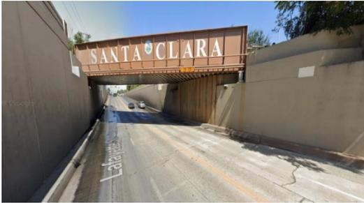
There is constant ponding of groundwater on Lafayette Street at the underpass located next to the Lafayette Street Subway Pump Station. The scope of work for the first phase of this project consists of evaluation of the existing site condition, which includes geotechnical boring and testing, structural analysis, and preparing schematic design plans and report.
