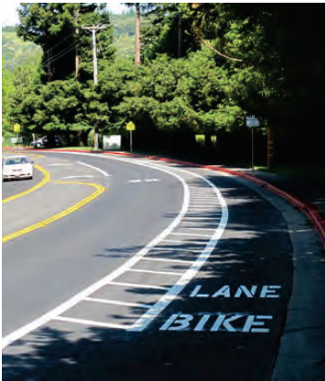
EXAMPLE OF BUFFERED BIKE LANES A buffer between vehicle traffic provides additional horizontal separation from vehicles.
