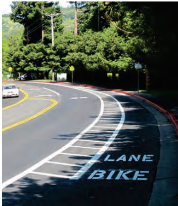
EXAMPLE OF BUFFERED BIKE LANES A buffer between vehicle traffic provides additional comfort for cyclists.
