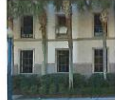
The landscaped portion of this setback is treated with the same quality of design as the rest of the building. Required and landscaped setback shall be maintained, and the landscaped setback shall be maintained.
