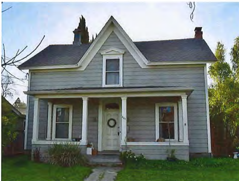
Top left: 1404 Lincoln Street. The gabled roof and the porch with square Doric posts suggest Greek Revival.
