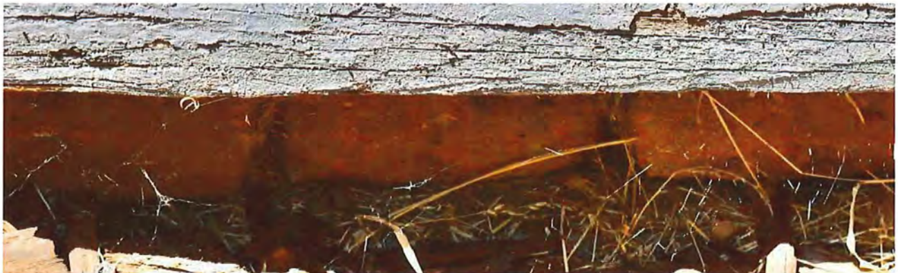
Below: The brick foundation.
