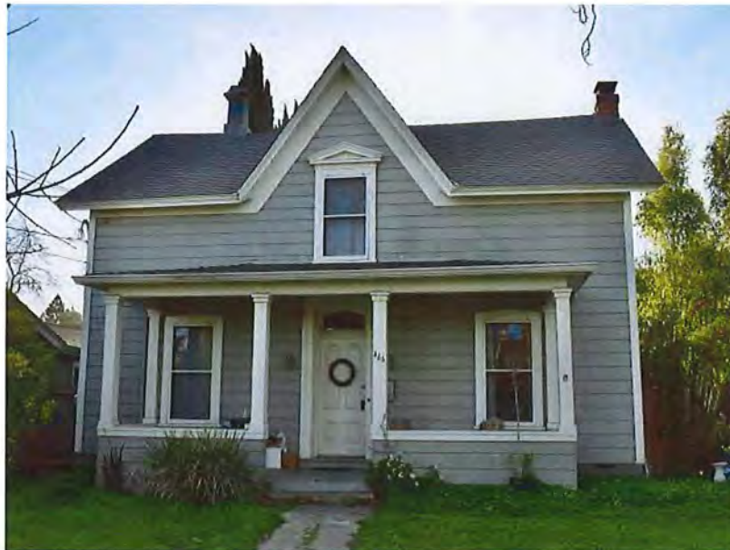
Top left: 1404 Lincoln Street. The gabled roof and the porch with square Doric posts suggest Greek Revival.
