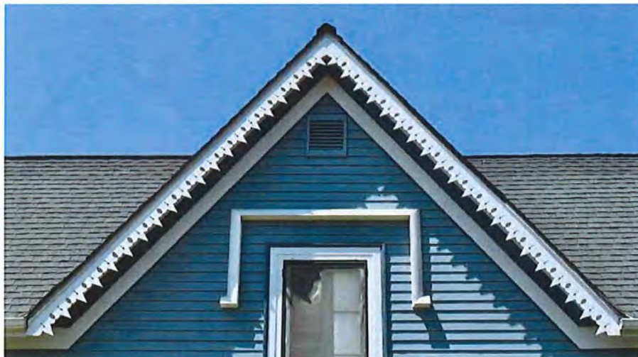
The front of the house with a detail of the bargeboard and the drip mold over the second story window.
