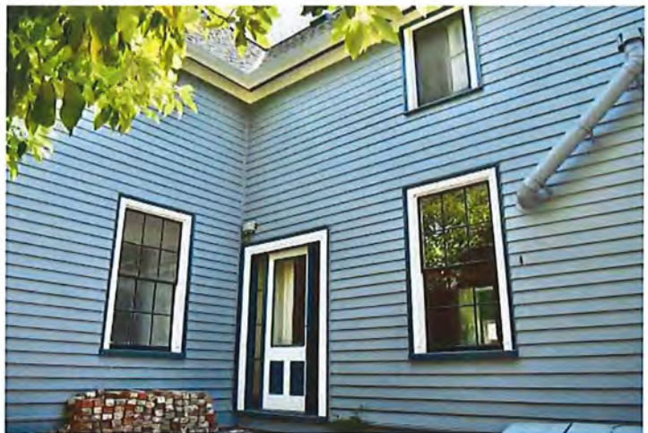
Below: View looking SE at the rear side of the front block and the north side of the rear stem.
