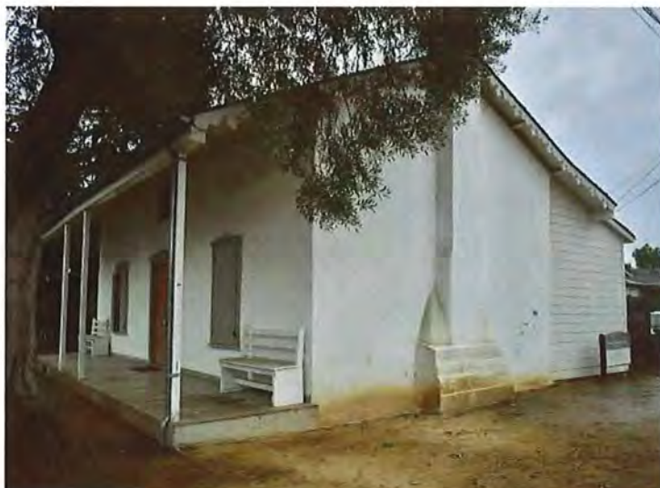
The Berryessa adobe, 373 Jefferson Street. It has been dated to the 1840s. Shallow-pitched pediments over the door and windows evoke the Greek Revival, while carved bargeboards in the gable are Gothic Revival.
