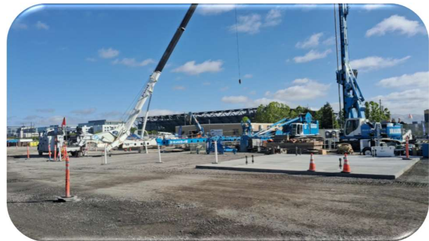
Assembly of BG-55 Drill Rig – In Preparation for Ground Improvement Work
