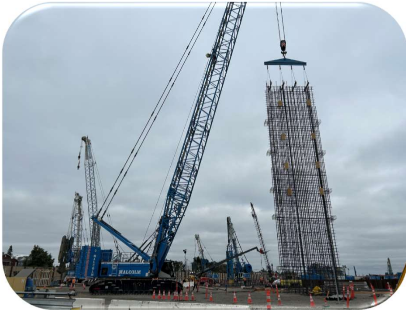
Rebar Cage Lift for D-Wall Construction
