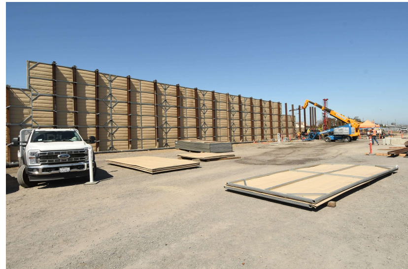
Temporary noise curtain installation adjacent to railroad tracks
