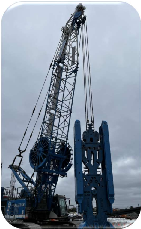
Slurry Wall Drilling Equipment – Hydraulic Grab Used to Excavate Material
