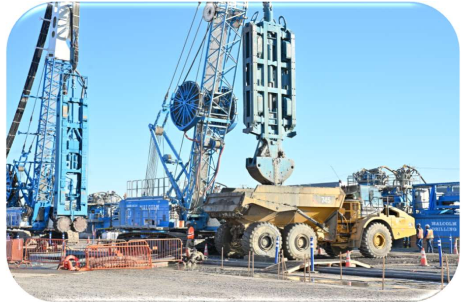
Spoils from D-Wall Excavation to be Off Hauled to Muck Bins
