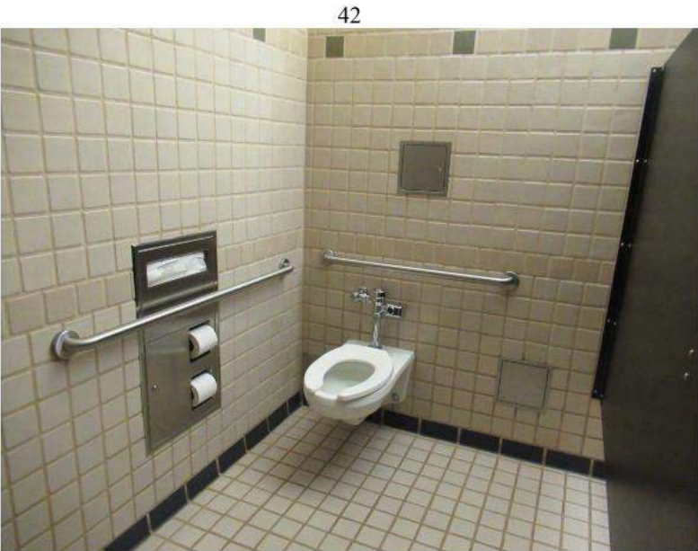
42. Toilets have automatic flush valves.
