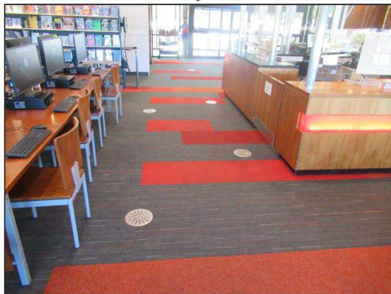
3. The entire floor area is raised flooring with vents for air circulation.
