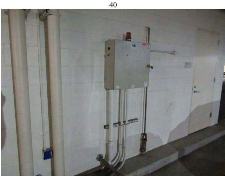
40. Controller for one of the sump pumps in the garage level.
