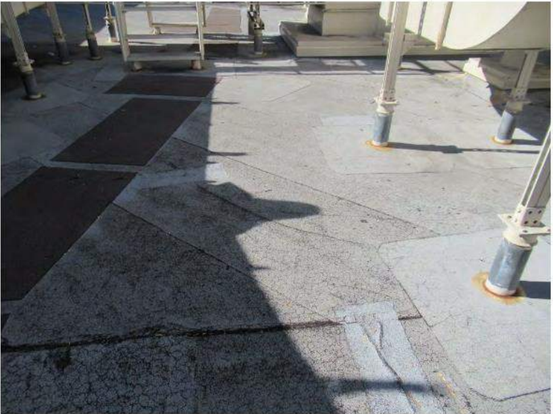
22. Membrane is original installed in 2004.
