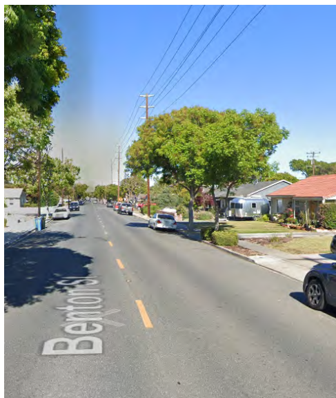
PHOTO: EXISTING CONDITIONS ON BENTON
