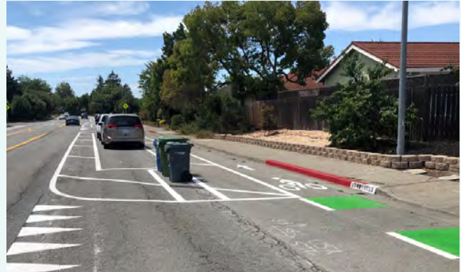
Designated trash bin locations at driveways on the Rainier Avenue Paving and Traffic Calming Upgrades Project, City of Petaluma, CA
