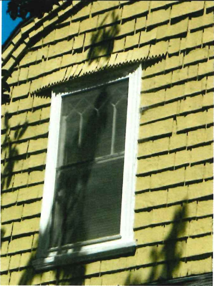
Photo No: 100_2358 View: Front facade & South side-elevation second story windows with curved row of shingles that have saw-tooth ends & lattice muntin enhanced beveled glass panes in upper sashes. Photo Date: May, 2018; Camera Facing: NE
