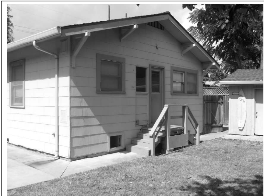
Photo 7: View of the rear façade.
