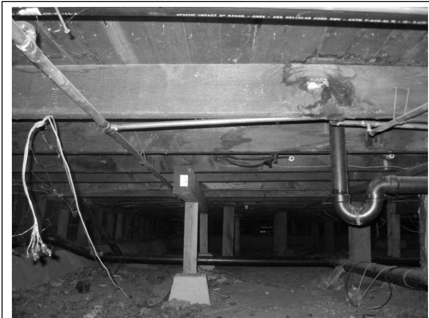
Photo 10: View of the crawl space and support beams.
