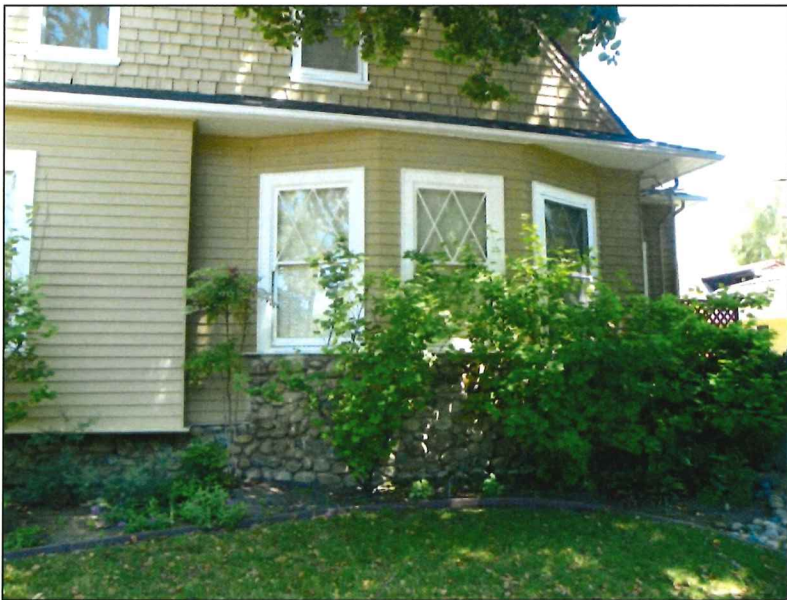
Photo No: 100_2363 View: South side-elevation showing first story bay and cobblestone sheathing Photo Date: May, 2018; Camera Facing: N
