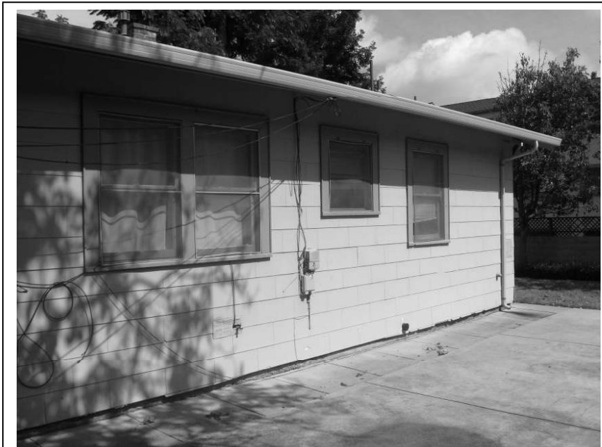
Photo 9: View along the southern façade from the west.
