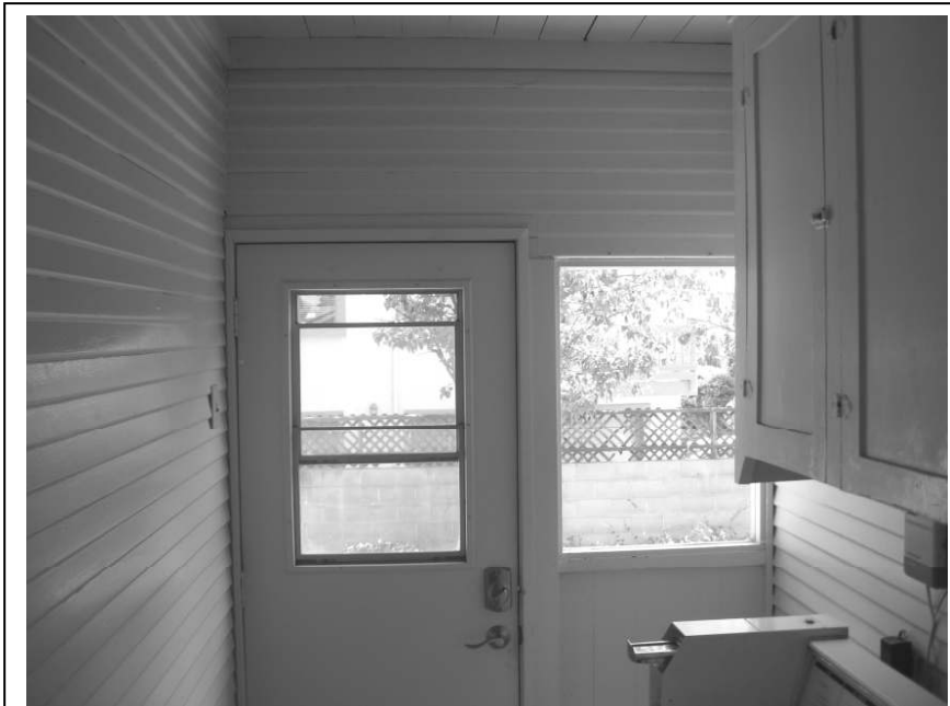
Photo 14: View of the laundry area, likely an enclosed porch.
