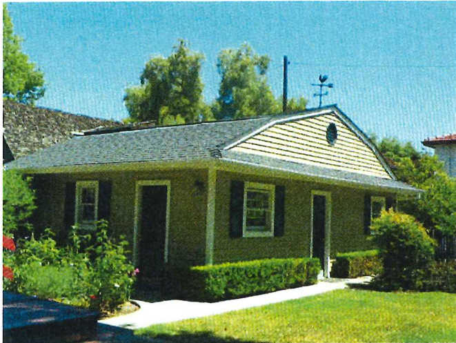
Photo No: 100_2375 View: Detached garage with office space (not original) Photo Date: May, 2018; Camera Facing: N
