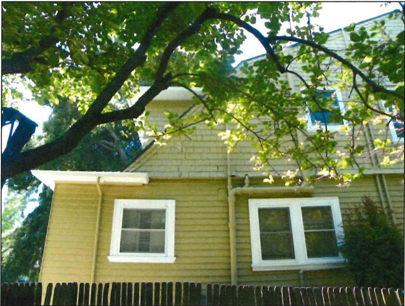
Photo No: 100_2344 View: Partial North side-elevation showing rear enclosed porch and upper projecting gable Photo Date: May, 2018; Camera Facing: SE
