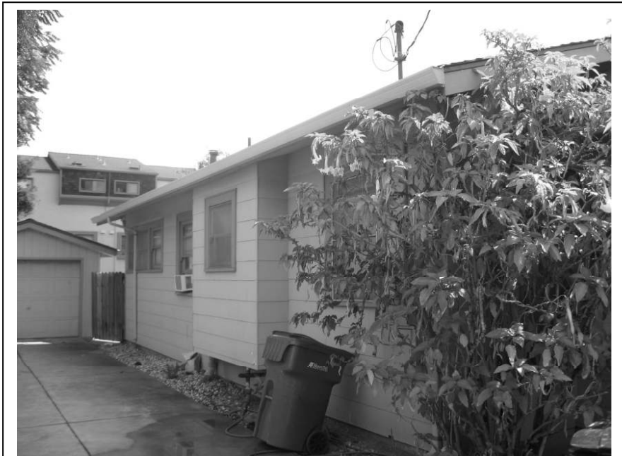
Photo 5: View along the northern façade.
