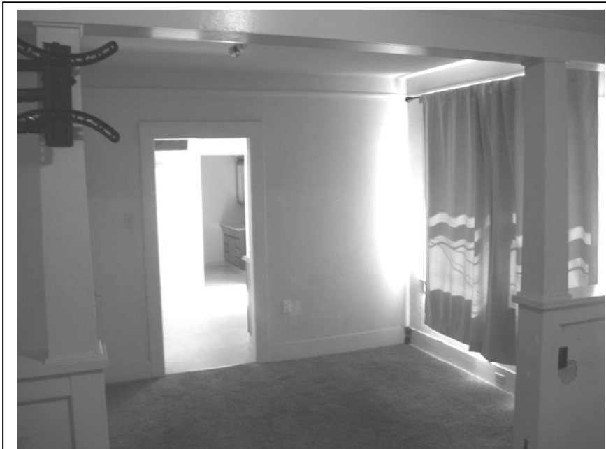
Photo 11: Interior view of the front room showing columns.
