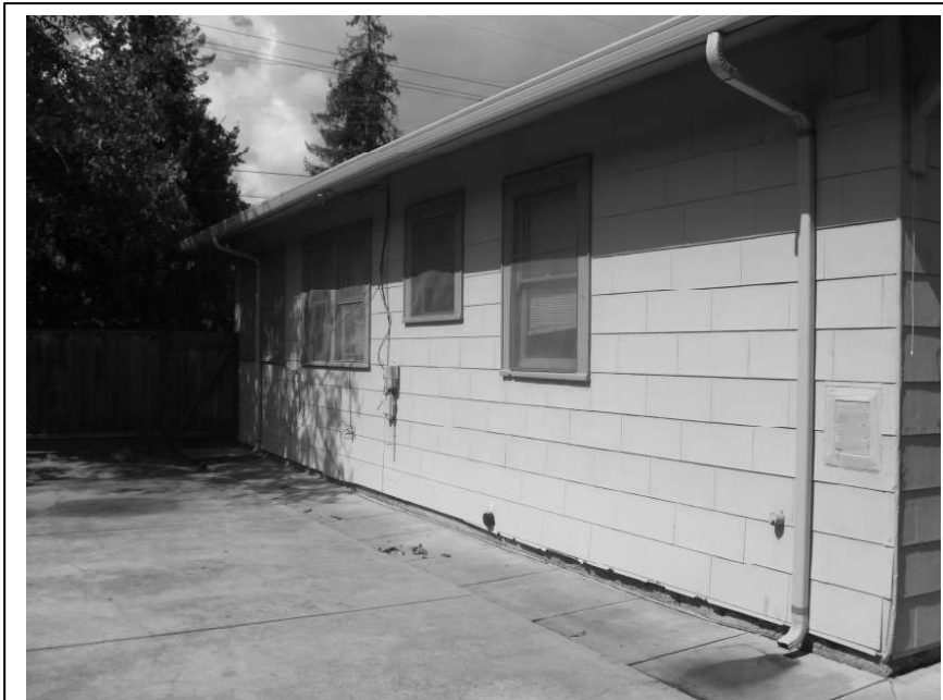
Photo 8: View along the southern façade from the east.
