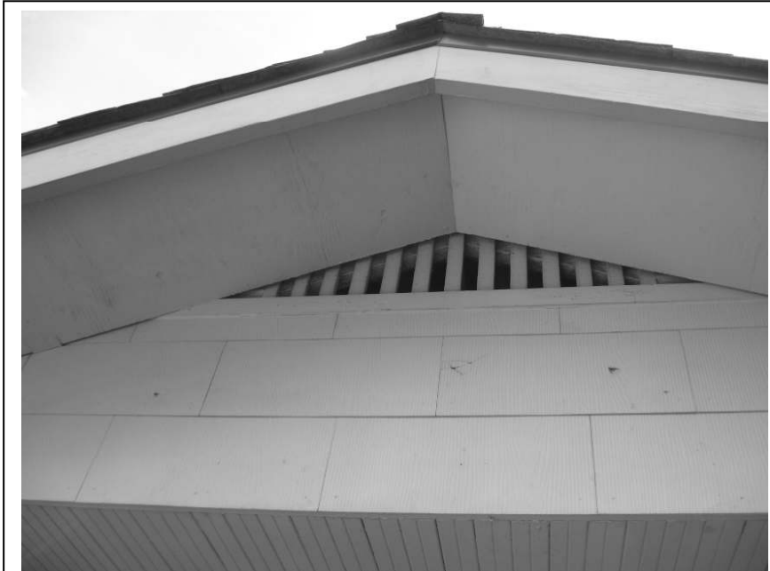
Photo 3: Detail of small vent at the top of the porch gable.
