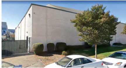
E3 - EXISTING EAST YARD AND NORTHEAST CORNER OF BUILDING B
