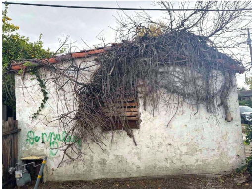
Photograph 2: 520 Hilmar St, northeast elevation, camera facing southwest, November 13, 2024.
