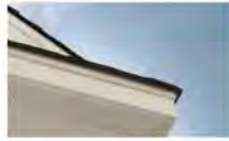
James Hardie Soffit Fiber Cement Vented Smooth Panel painted black satin finish 2X10 FASCIA JAMES HARDY - WITH ROYAL MOLDING
