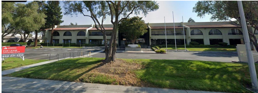
Existing 2-story office building
