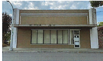
MONROE ST @ FRANKLIN ST ART DECO SHOPFRONT
