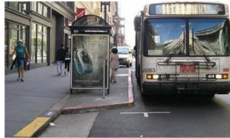
Bus Bulb in San Francisco Source: National Association of City Transportation Officials
