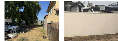
EXISTING WALL ON ALVISO FRONTAGE. EXAMPLE OF PROPOSED 6 FT HIGH MASONRY WALL, COATED WITH STUCCO
