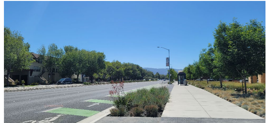
Figure 1819: Conceptual Graphic of Before and After Implementation of Elevated High-Capacity Transit System, West of I-280
