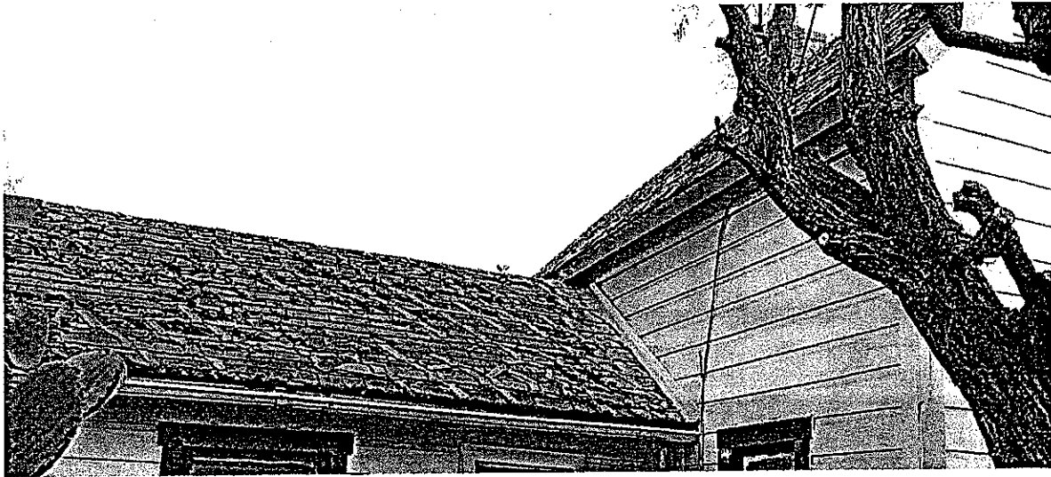
Figure 6: Roof at left side of structure
