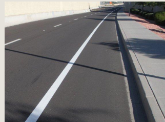
Edgelines and Centerlines (install or modify)
