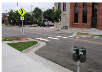
Curb Extensions/Bulb-outs, Curb Radius Reduction
