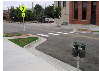
Curb Extensions/Bulb-outs, Curb Radius Reduction
