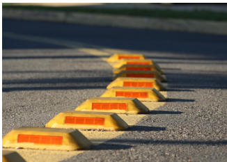
Raised Pavement Markers
