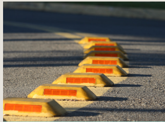
Raised Pavement Markers
