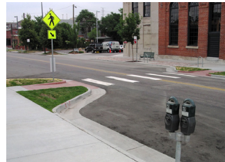
Curb Extensions/Bulb-outs, Curb Radius Reduction
