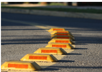
Raised Pavement Markers
