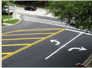
Upgrade Intersection Pavement Markings
