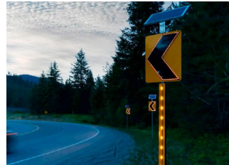
Improved Signage and/or Reflective Strips
