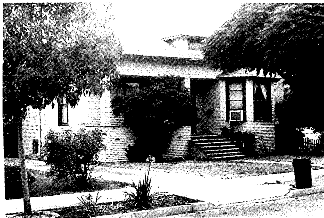
Front façade of 1226 Jackson Street, July, 1988. The photo appeared on the original historic inventory form. Front steps have since been reconstructed to add handrails.
