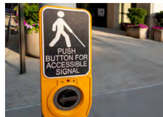
ADA Ramps & Audible Push Button Upgrades
