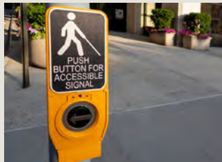
ADA Ramps & Audible Push Button Upgrades
