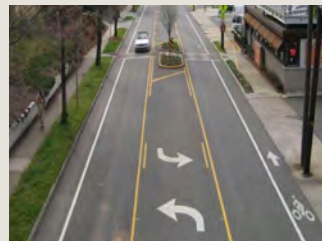
Two-Way Left-Turn Lane
