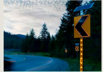
Improved Signage and/or Reflective Strips
