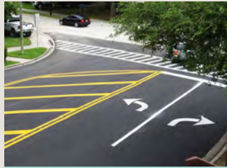
Upgrade Intersection Pavement Markings
