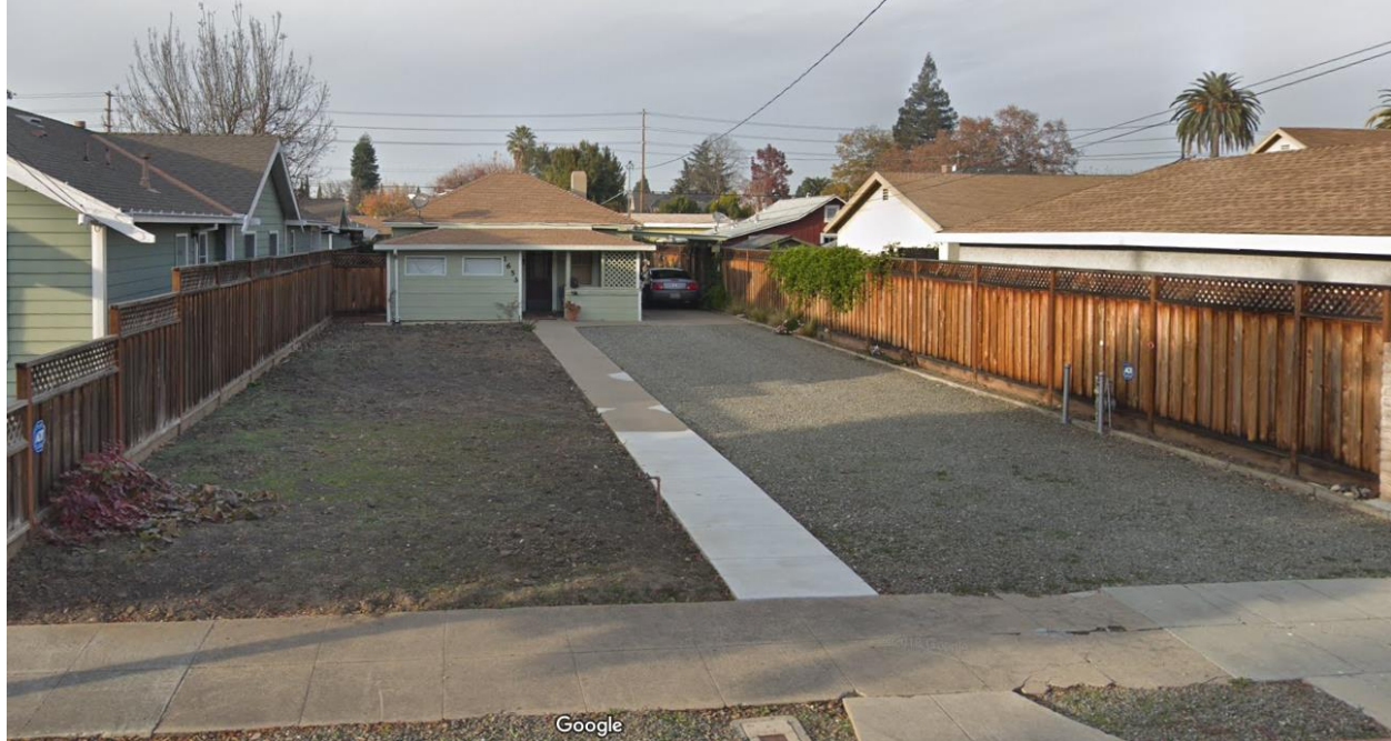
Front Elevation of 1653 Fremont Street:
