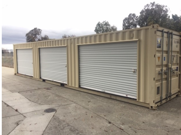
Storage Conex Garage for Apparatus allows for storage of three stadium vehicles in a lockable, weatherproof container.
