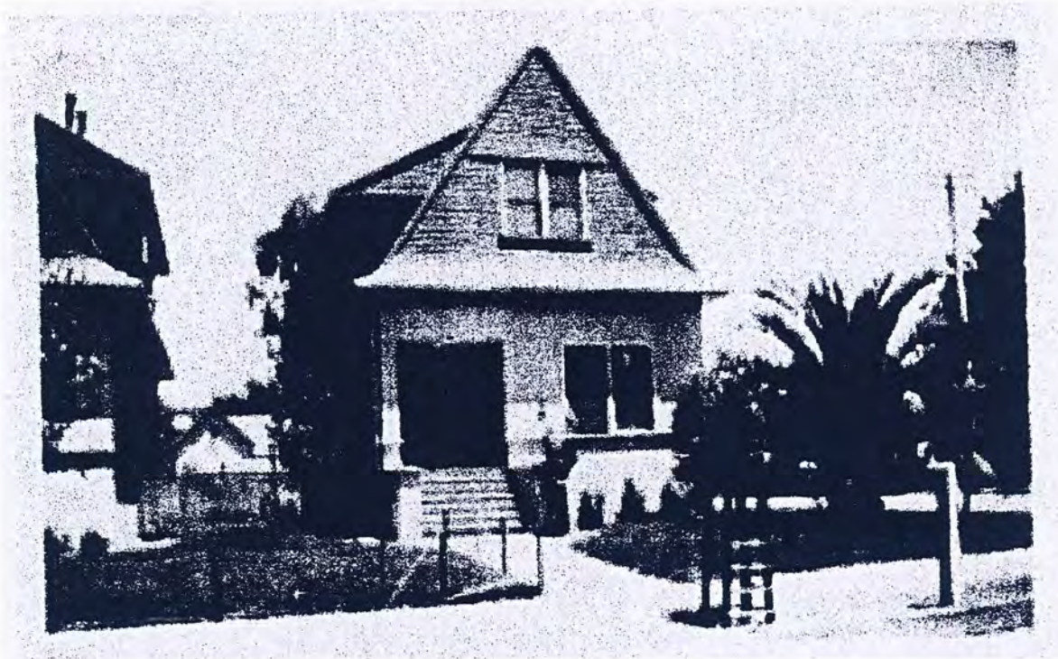
Taken in 1903-4, the above photo shows 811 Monroe Street, shortly after it was constructed.
