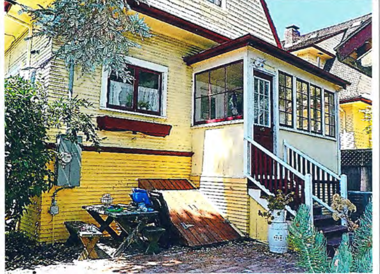
Photo No: 100_3253 View: Rear Façade showing sun porch, rear entry & basement entry Photo Date: 8/18/2023; Camera Facing: W
