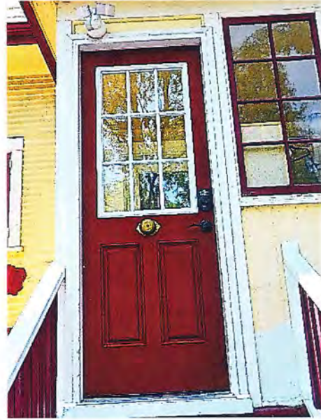
Photo No: 100_3268 View: Rear Door Photo Date: 8/18/2023; Camera Facing: E
