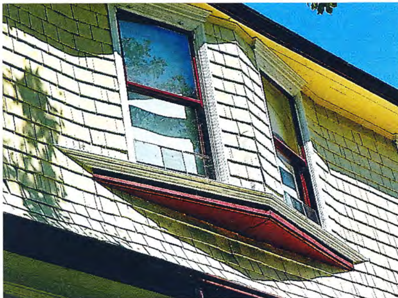
Photo No: 100_3249 View: S side-elevation Dormer - Triangulat Bay showing windows topped with an Architrave. Photo Date: 8/18/2023; Camera Facing: N
