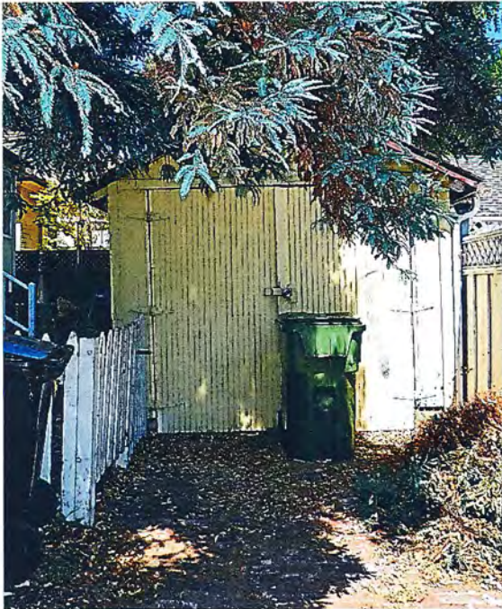
Photo No: 100_3255 View: Barage – Front Façade and brick driveway Photo Date: 8/18/2023; Camera Facing: NNW
