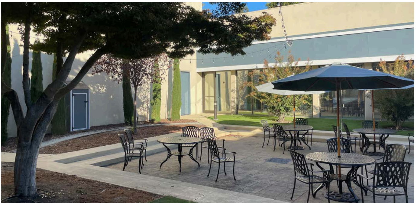
The Community Recreation Center courtyard is a space that could be redesigned to better serve residents' needs.
