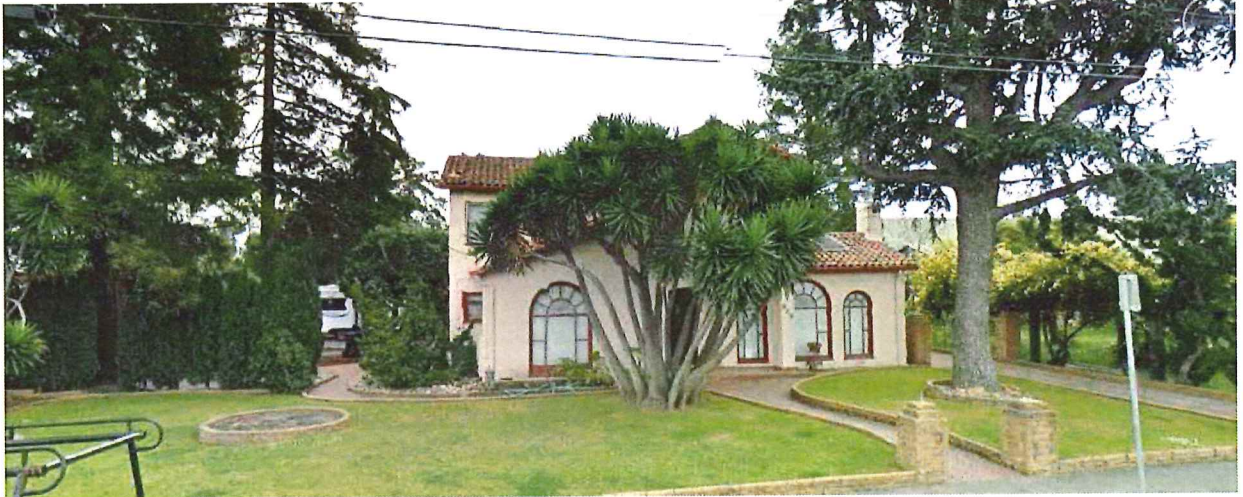
Photograph 1 820 Civic Center Drive.
