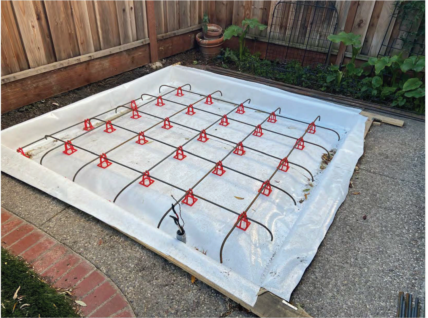
Stages of construction prior to neighbor complaint
