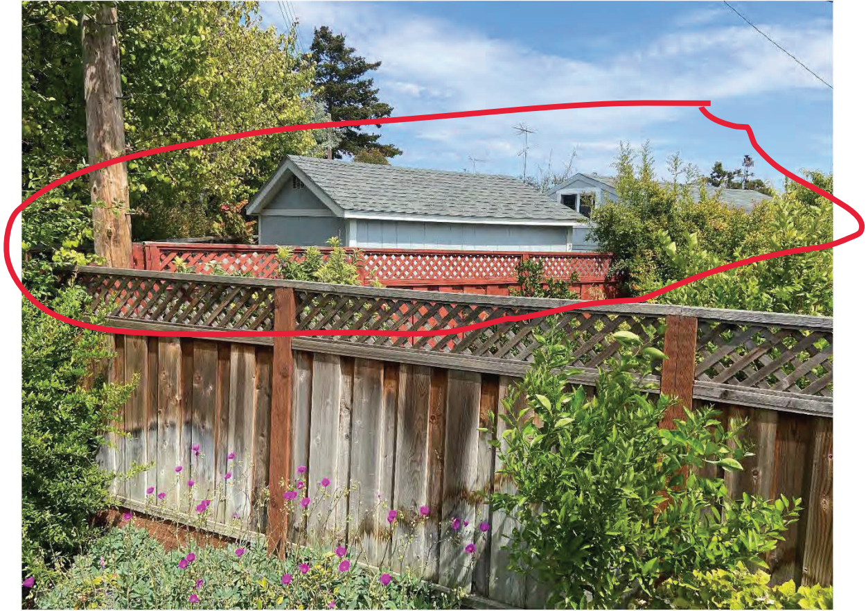
Non Code compliant sheds of 2361 Alberta Ct, visible from Back yard
