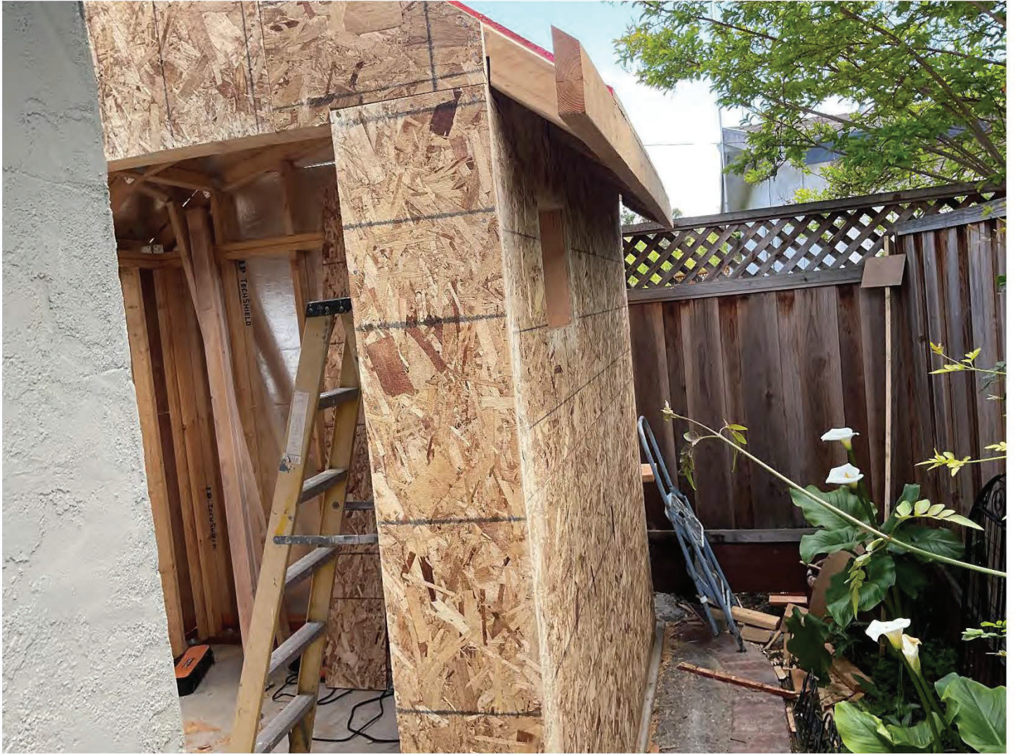
Stages of construction prior to neighbor complaint
