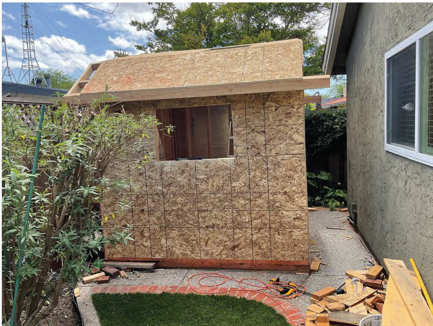
Stages of construction prior to neighbor complaint
