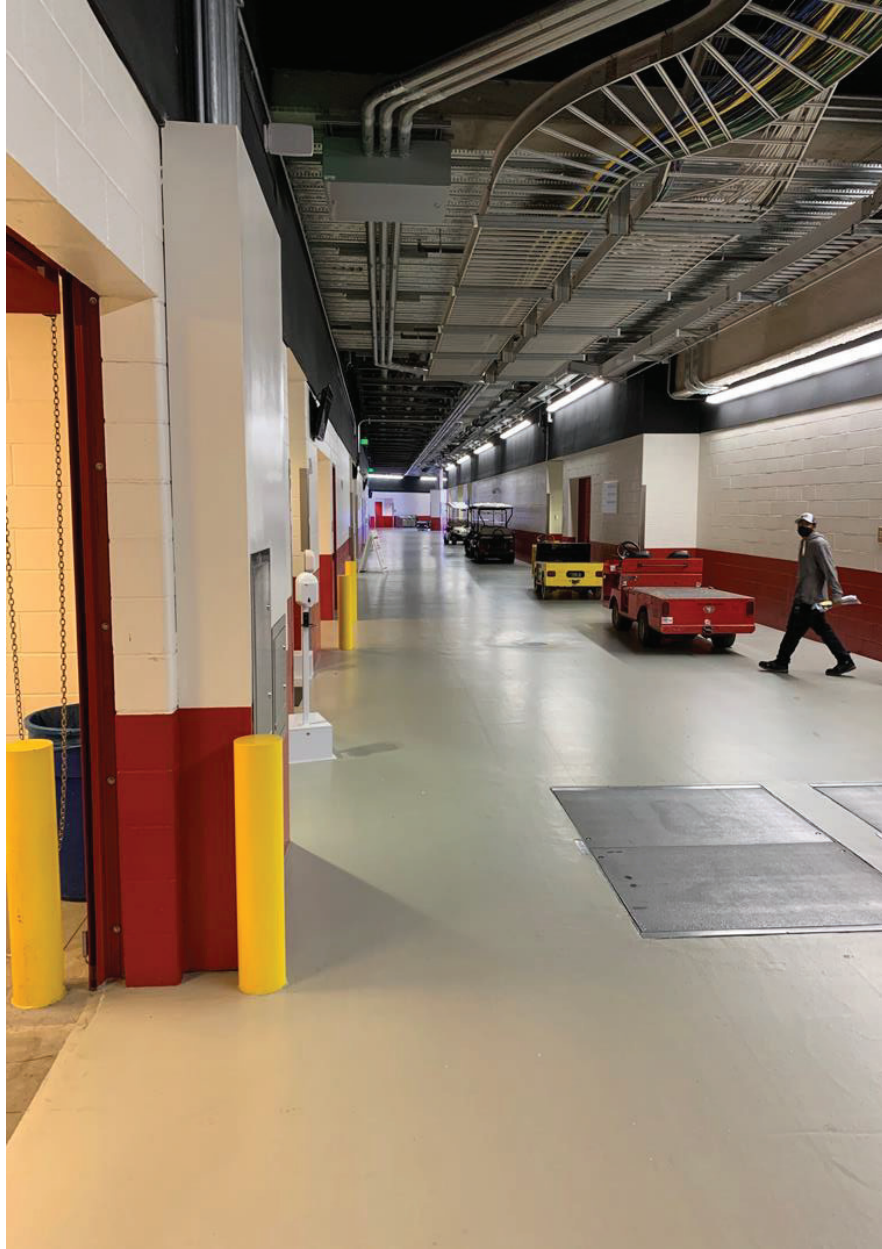
Figure 5: Photo of Corridor to Auxiliary Rooms (ALTERNATE #1 BID SCOPE) look into corridor tunnel area from field area.
