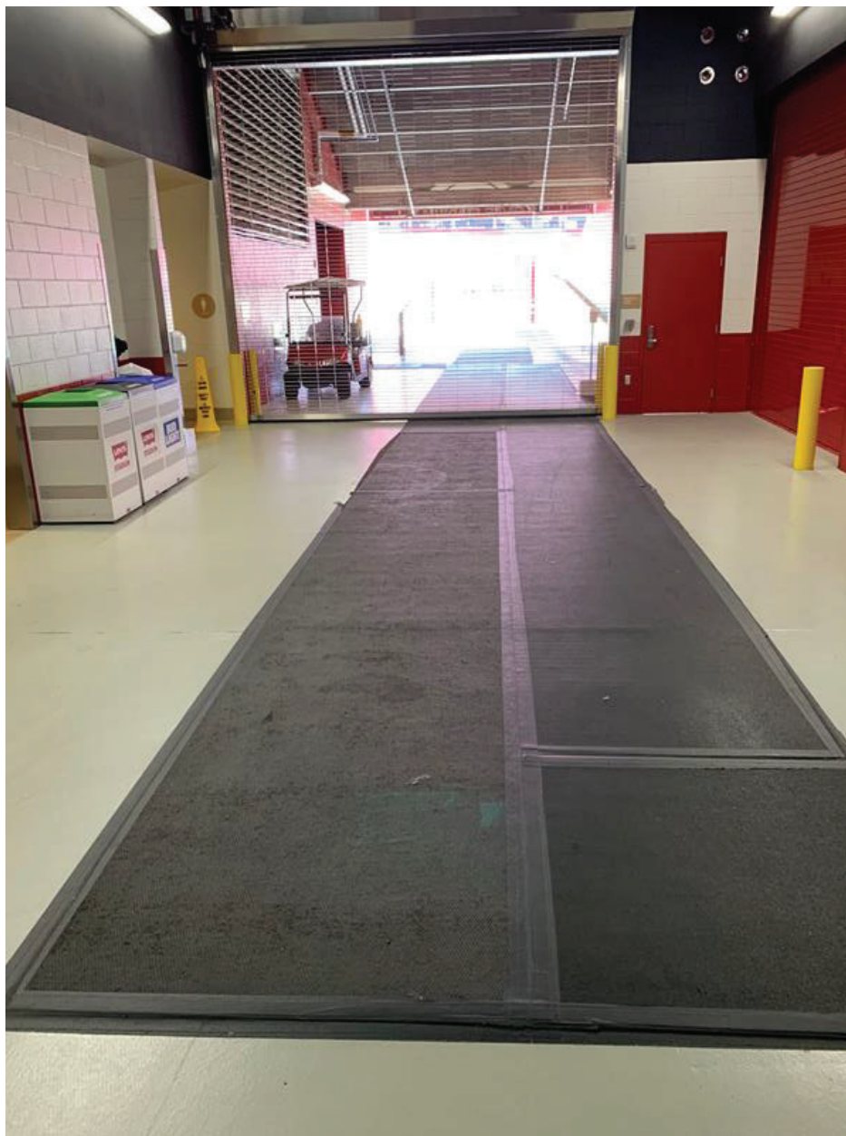
Figure 3: Photo of Northwest Tunnel (BASE BID SCOPE) look out to the field area.
