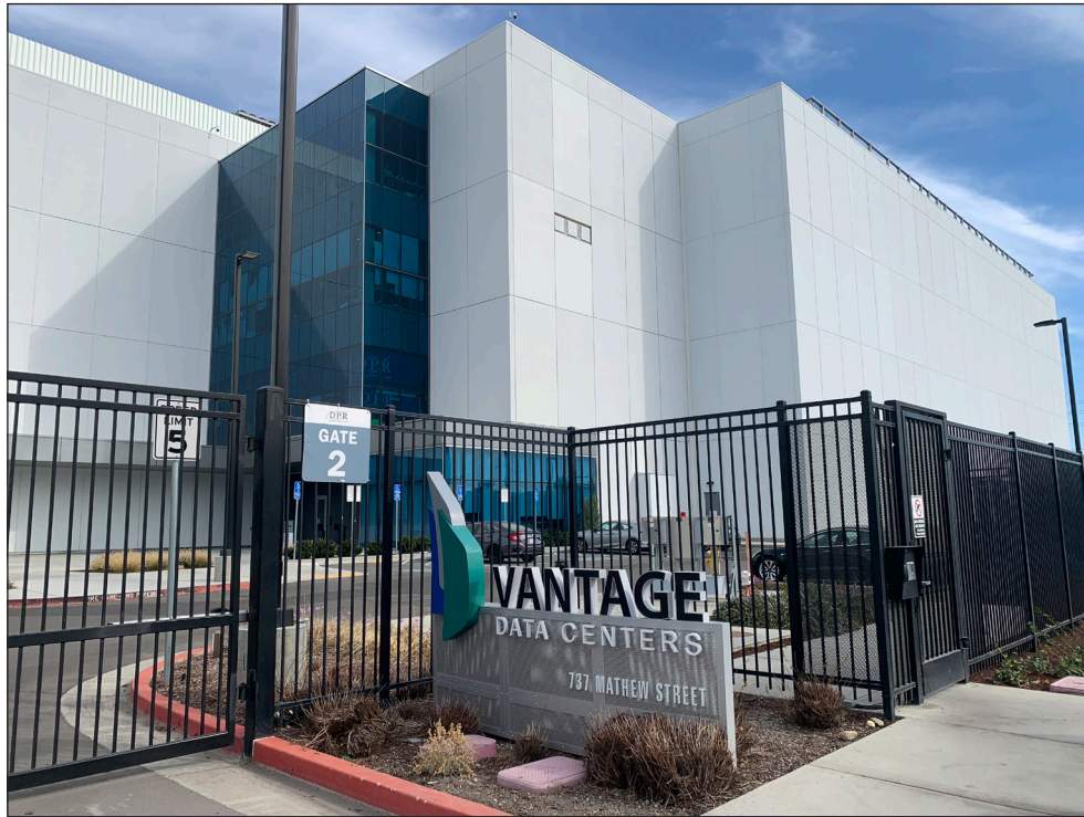
View A: View of Vantage Data Center facility looking northeast
