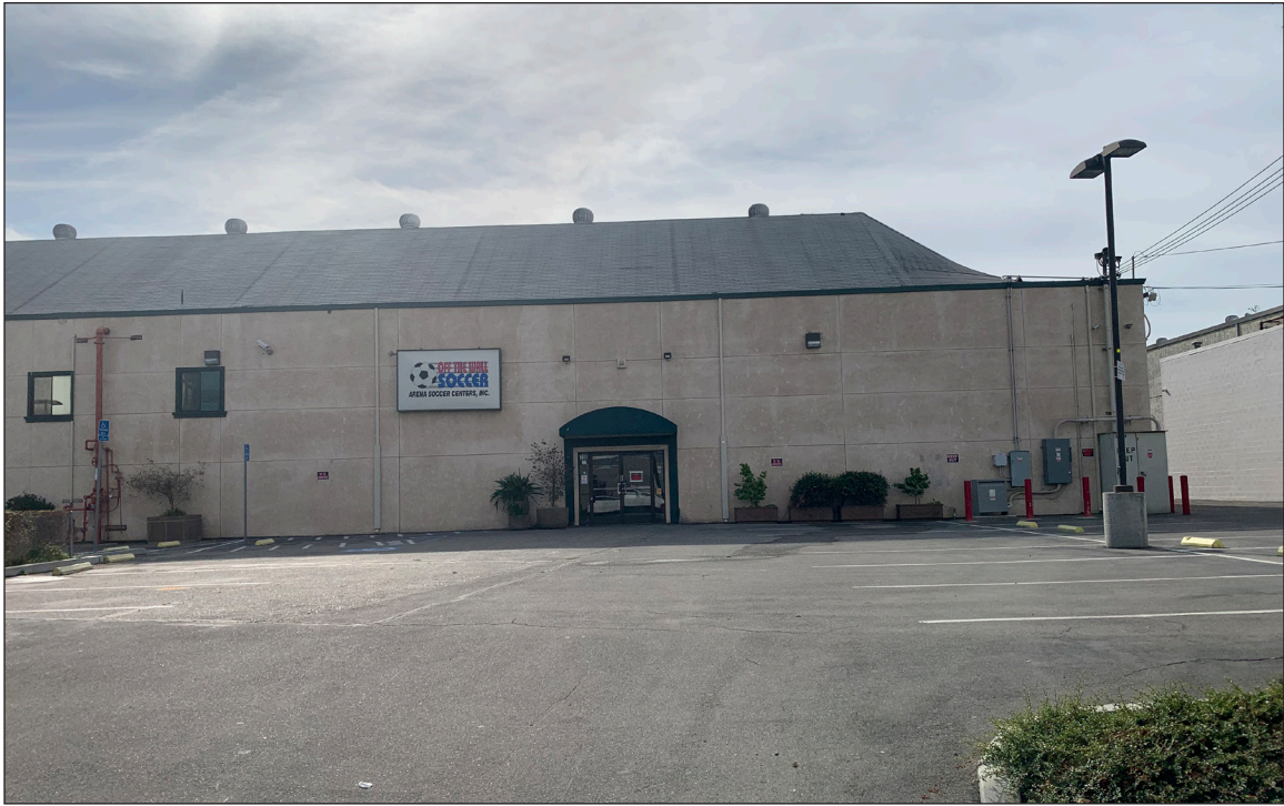
View C: Property located on the south side of Mathew Street looking southeast of 737 Mathew Street
