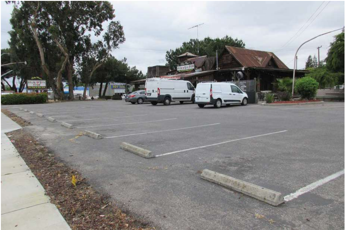
PHOTO 5: View of a restaurant building on Coleman Avenue looking north.
